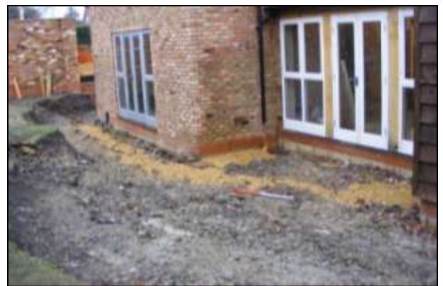
Plate 6: Ground reduction to the rear of the house
