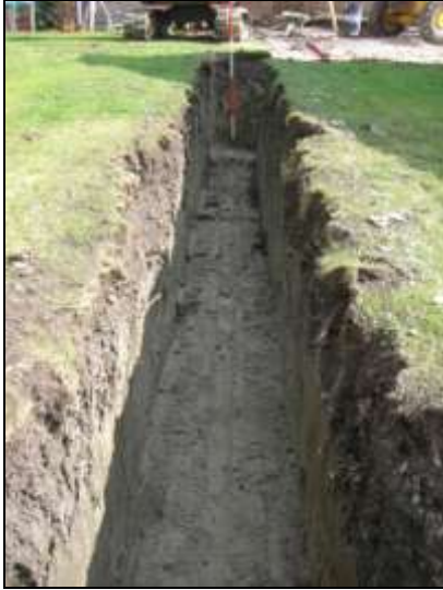
Plate 1: Trench to north of site, looking southeast. 2m scale
