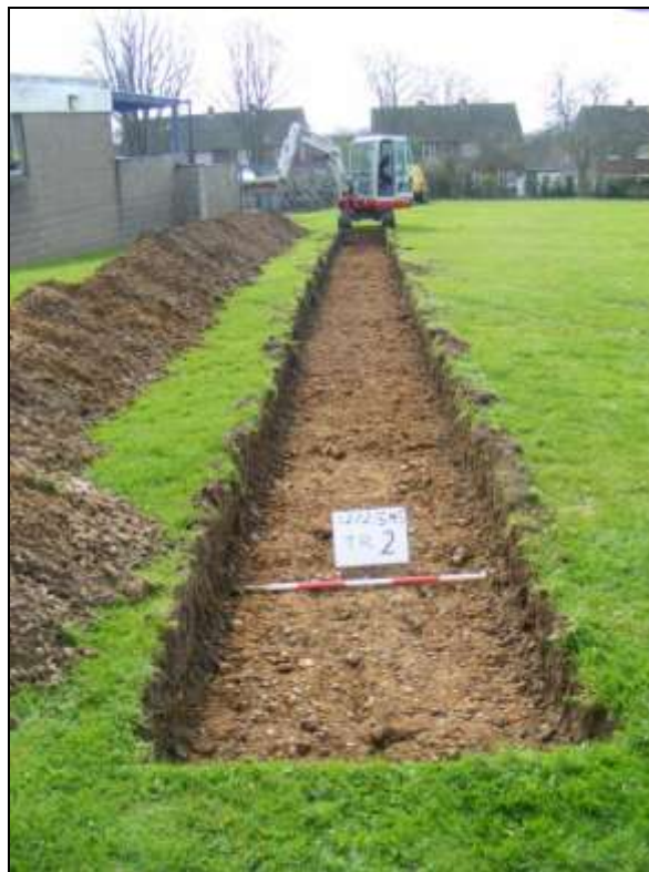
Plate 2: General view of Trench 2 looking southeast
