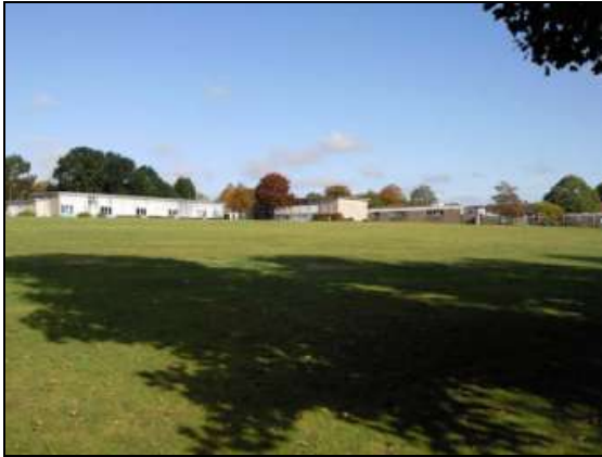
Plate 9: School complex, looking north
