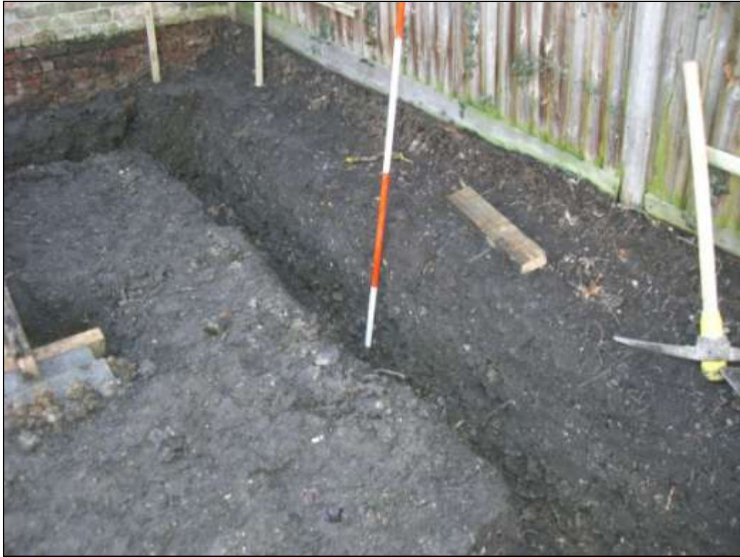
Plate 1: North-west footing trench, looking south-west
