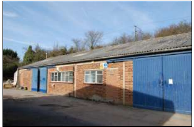
Plate 14: Building 2: south elevation, west end
