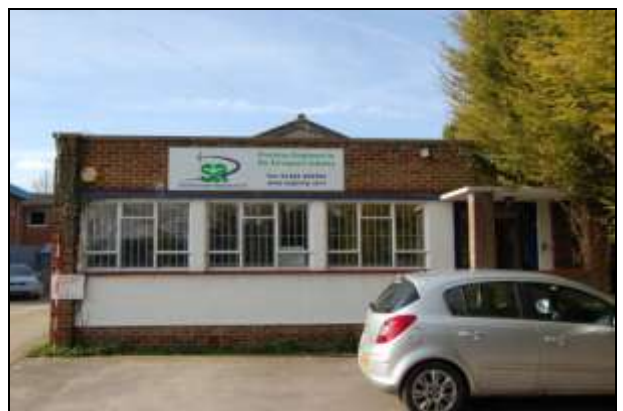
Plate 12: Building 2: east end
