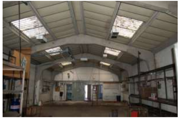
Plate 10: Building 1: industrial unit looking north
