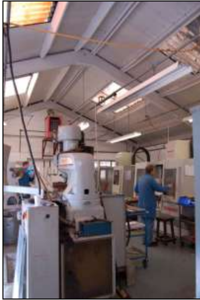
Plate 19: Building 2: western workshop looking northwest
