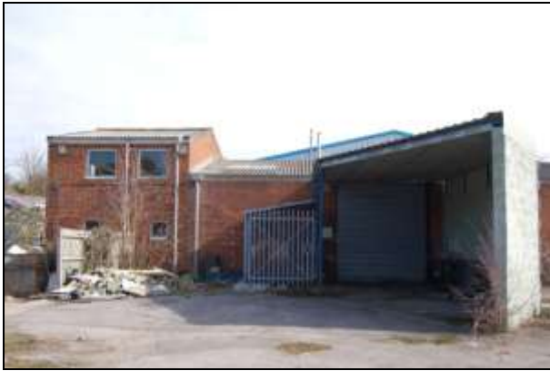
Plate 7: Building 1: west elevation, north
