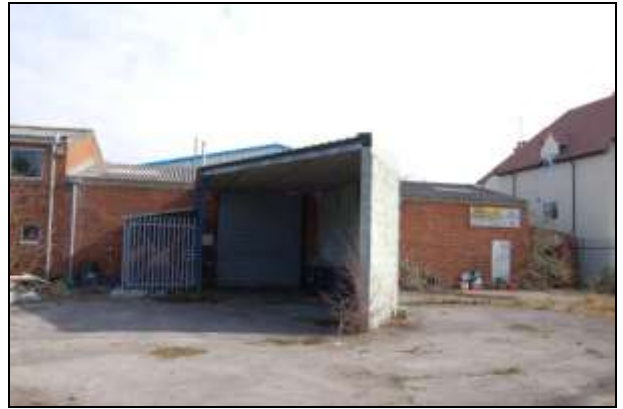
Plate 8: Building 1: west elevation, south
