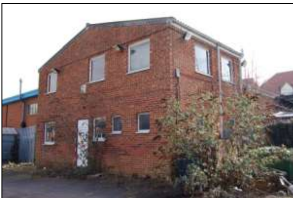
Plate 5: Building 1: north and west elevations
