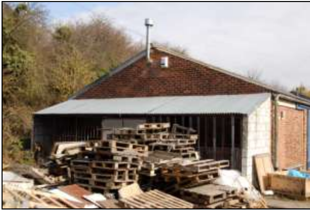
Plate 13: Building 2: west end
