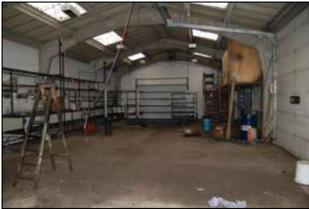
Plate 9: Building 1: industrial unit looking south
