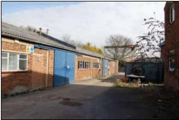
Plate 15: Building 2: south elevation, east end
