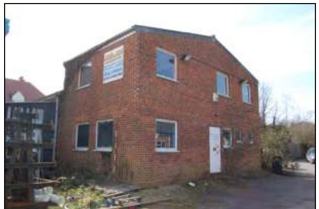
Plate 6: Building 1: north and east elevations
