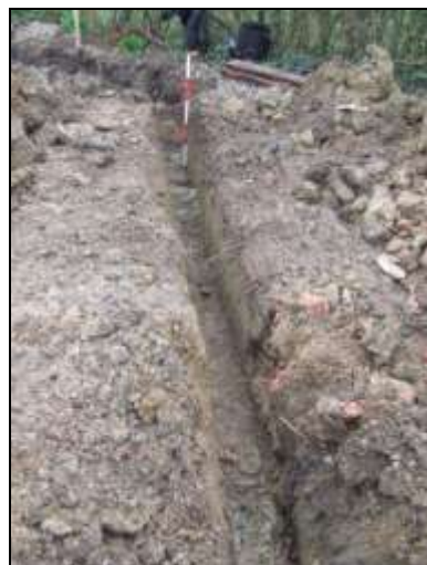
Plate 3: Service trench extending into driveway, looking south east ( scale= 1m )
