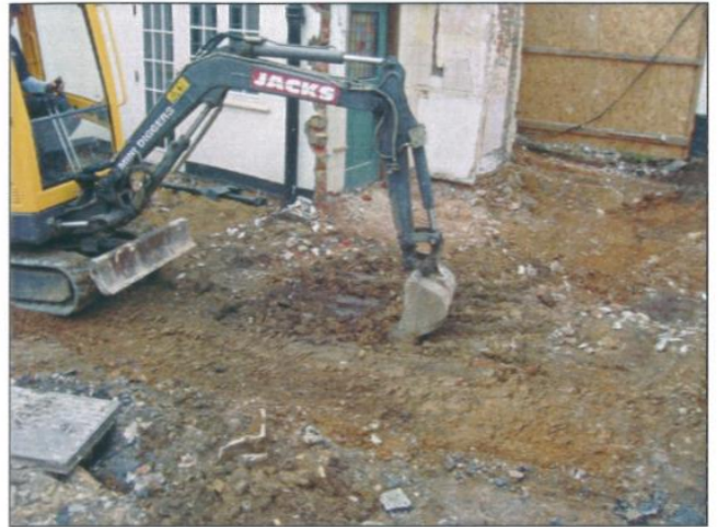
Plate 2: Final site clearance looking south
