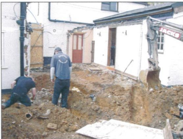
Plate 5: Drainage trenches looking south west
