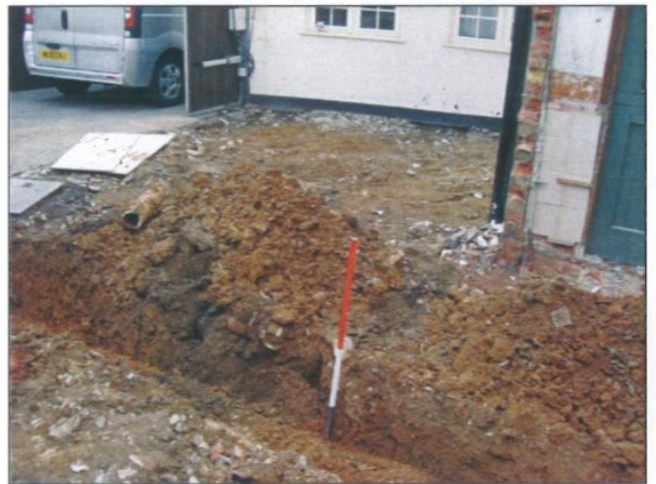
Plate 4: North west facing section of drainage run
