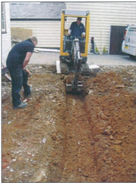
Plate 3: Excavation of drainage run looking south
