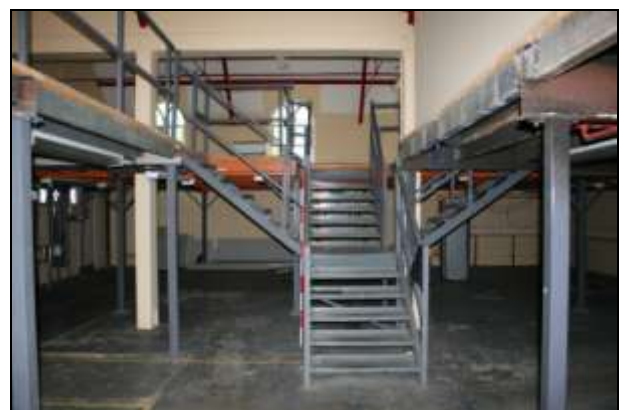
Plate 16: G3, central stairs, view south
