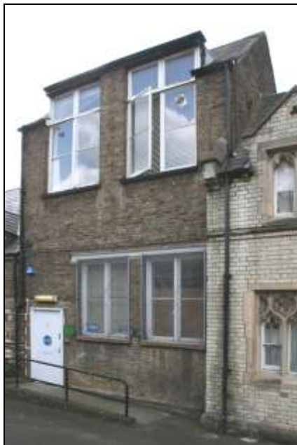
Plate 5: Link building: north elevation, from north
