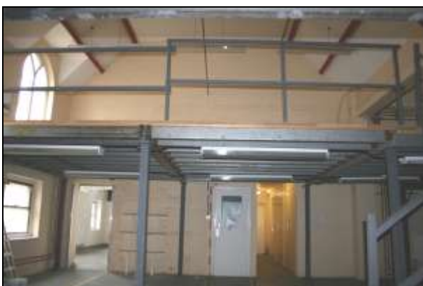
Plate 15: G3, north-east quarter, view east (full height)
