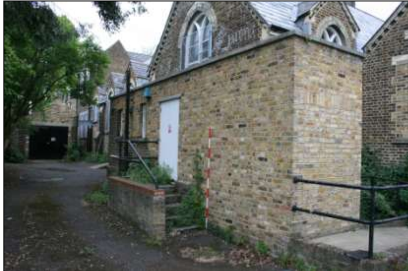
Plate 8: School: south-east corner, from south-east
