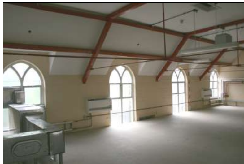
Plate 20: F1, south aisle, view south-west
