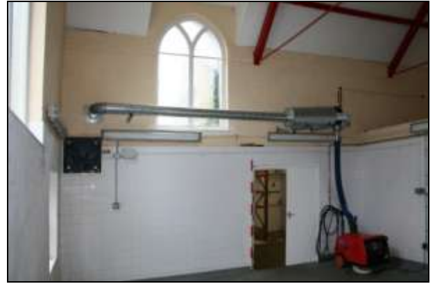
Plate 22: G4, view south-east
