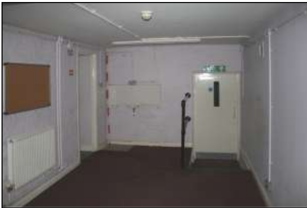
Plate 29: G9, view south-west
