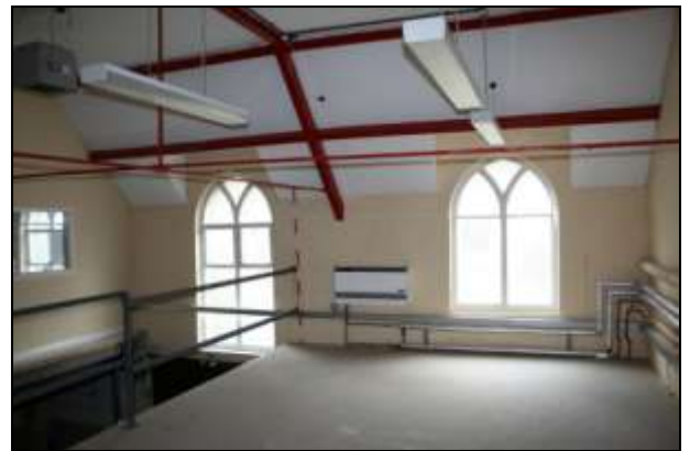
Plate 18: F1, north aisle, view north-west
