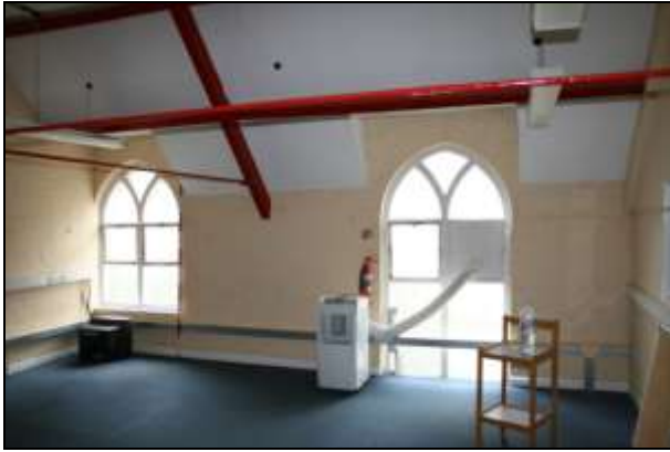
Plate 21: F2, view north-west
