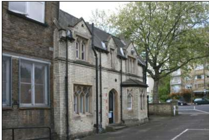
Plate 2: Cottages: north elevation, from north-east
