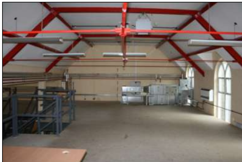
Plate 19: F1, south aisle, view east
