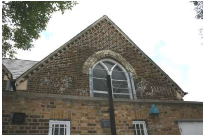
Plate 9: School: detail of south-east gable, from south
