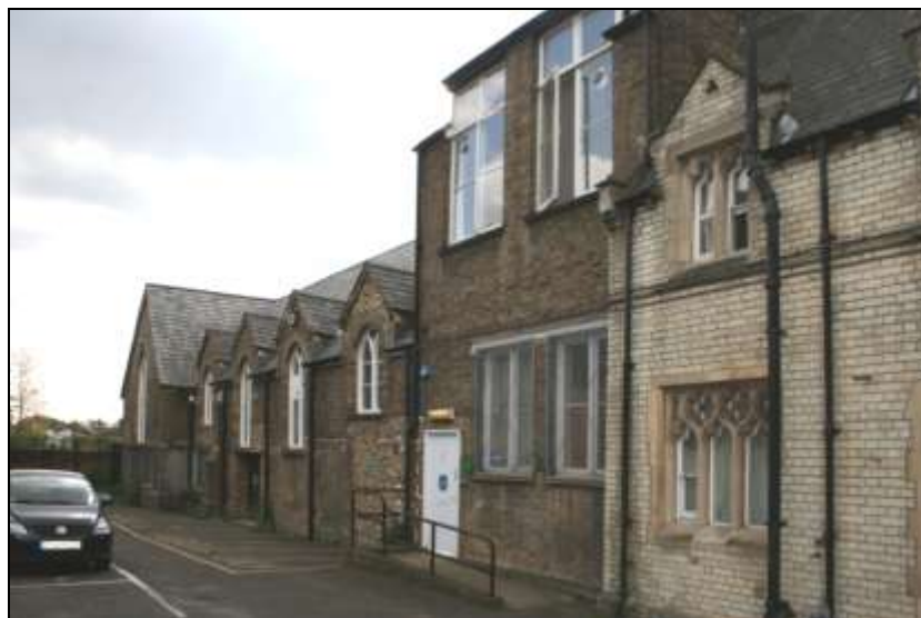
Plate 3: North elevation, general shot from north-west
