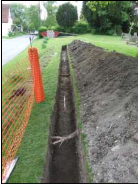
Plate 7: Drainage trench 2, looking SW (scale 2x1m)
