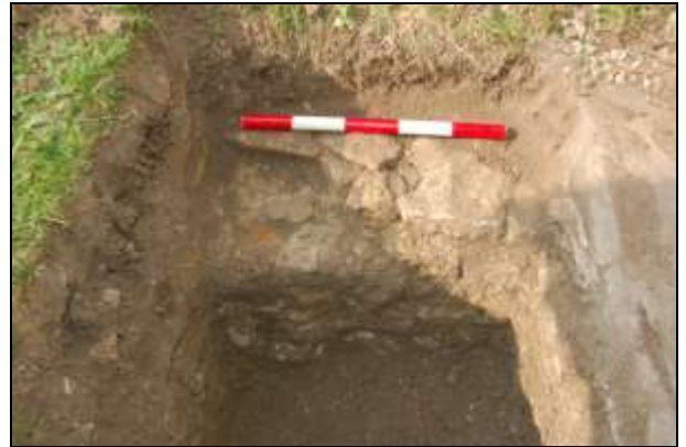
Plate 2: Inspection Chamber: Wall and floor surface (scale 500mm)
