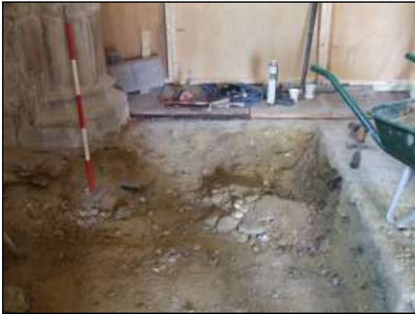
Plate 1: New WC and Tea Port Area (scale 1m)
