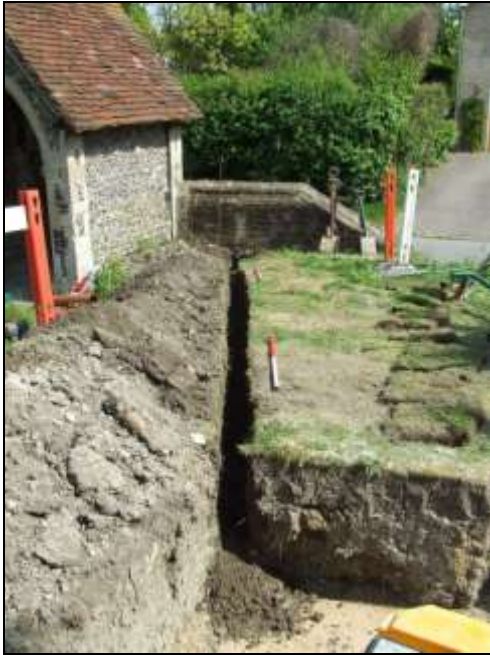
Plate 11: Drainage trench 3, looking SE (scale 2x1m)
