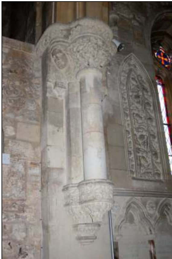
Plate10: Chancel arch detail
