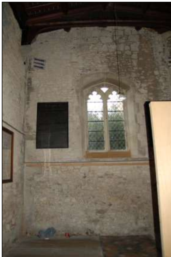
Plate 4: South end of west wall
