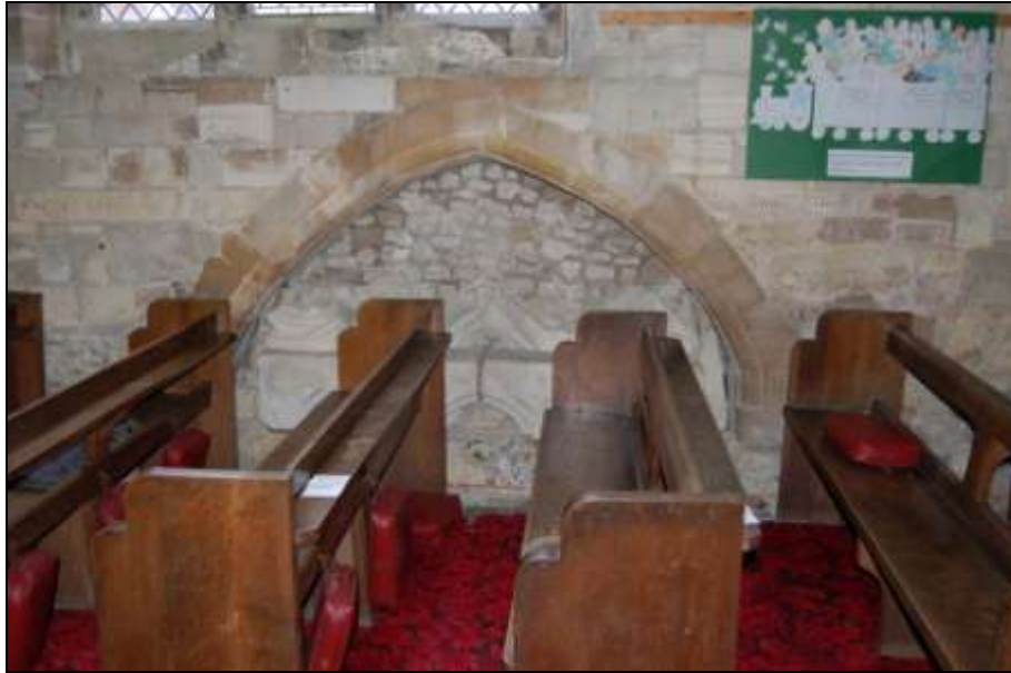
Plate 15: Arch in south aisle
