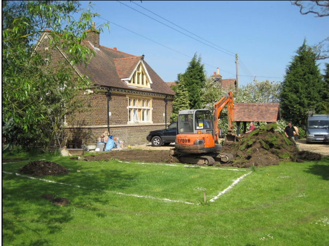
Plate 1: View NW across site of proposed new building
