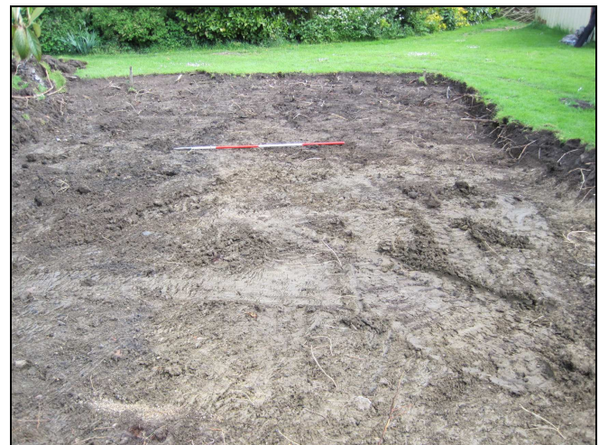
Plate 4: Looking NE across reduced ground level of new garage
