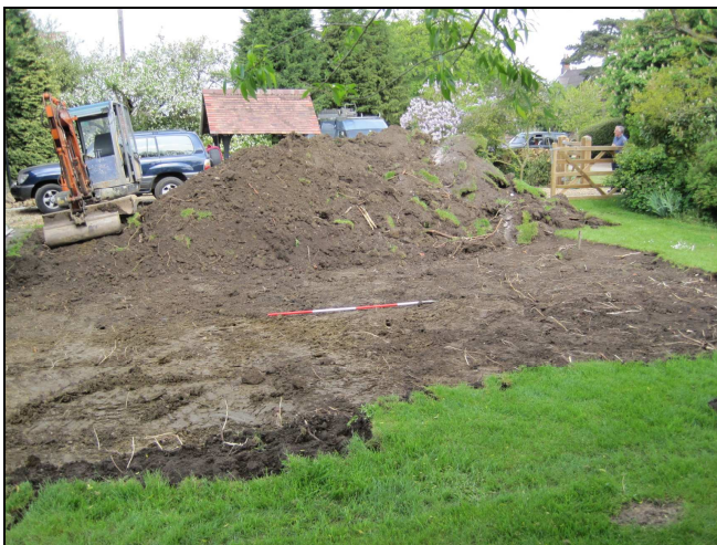
Plate 3: Looking NNW across reduced ground level of new garage
