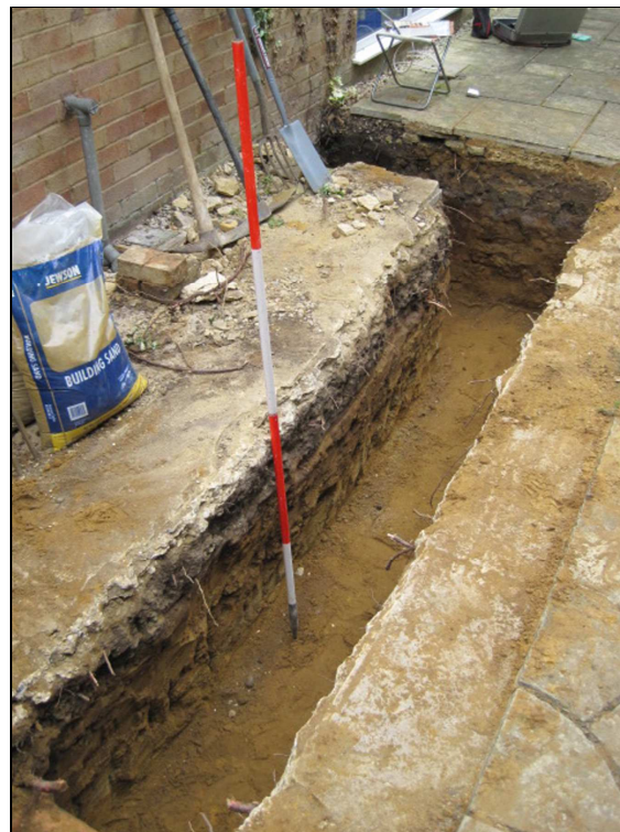
Plate 3: North-facing section of footing trench, looking south-west
