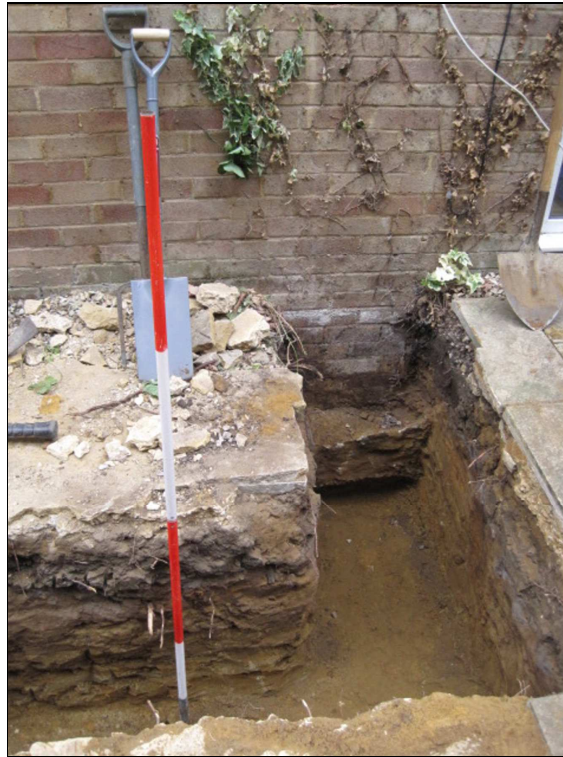
Plate 2: West end of footing trench, looking south
