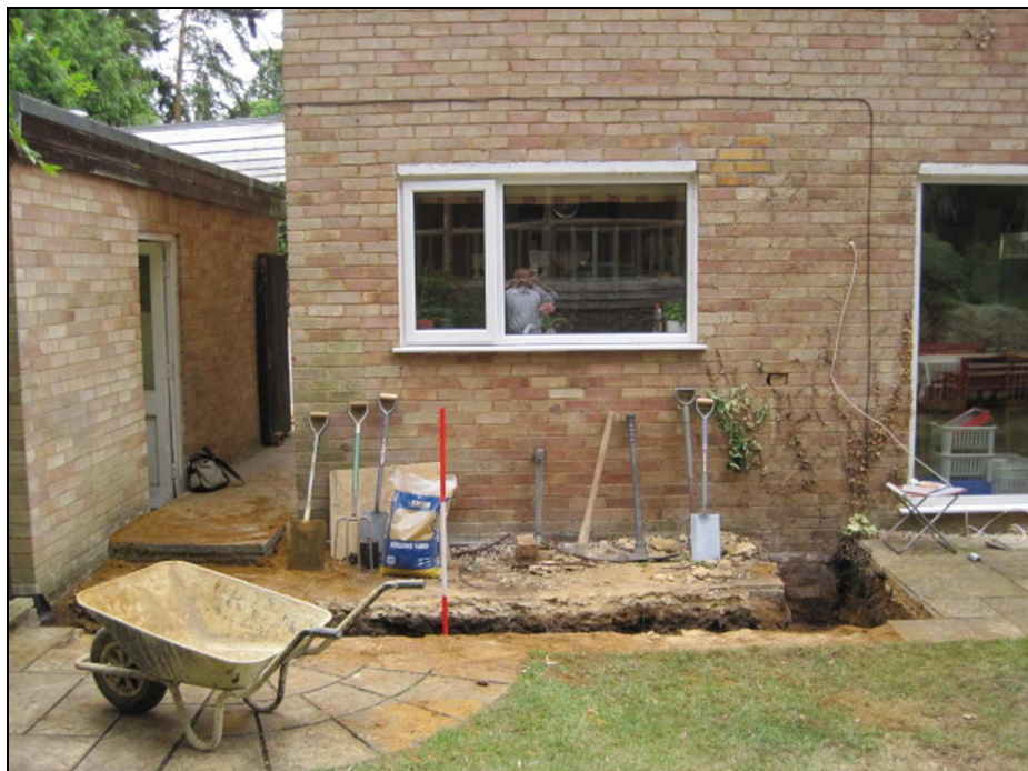
Plate 1: Location of footing trench, looking south
