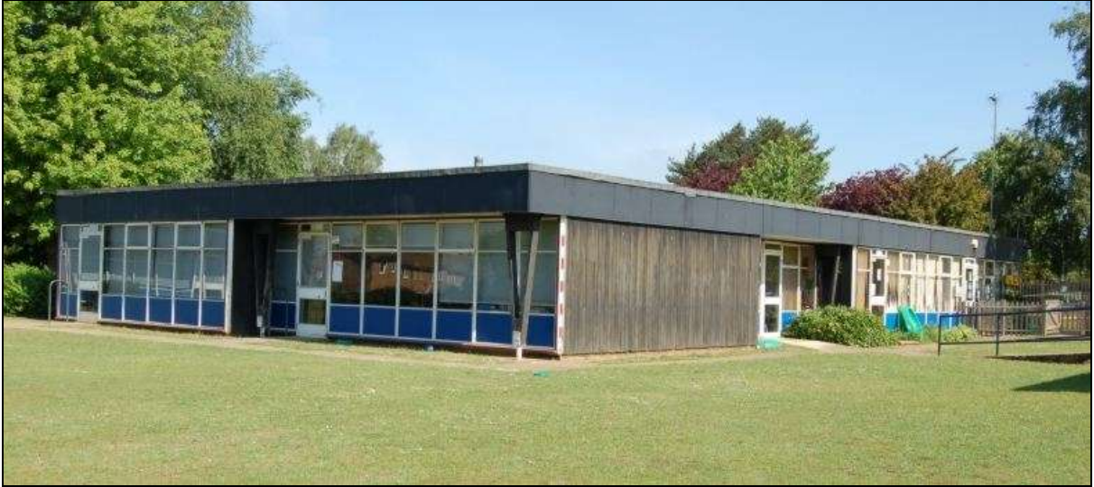
Plate 1: Block B, south-east corner from south-east
