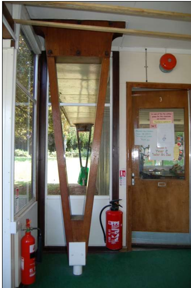
Plate 4: Block E, corridor (145), example of Y pillar, looking east
