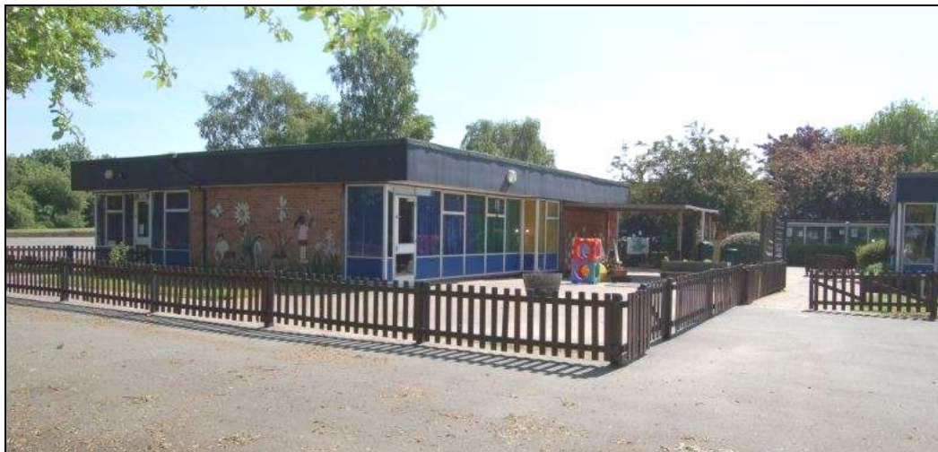
Plate 25: Block F, south-west corner from south-west
