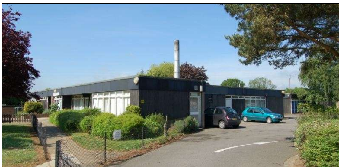
Plate 5: Block A, north-east corner from north-east
