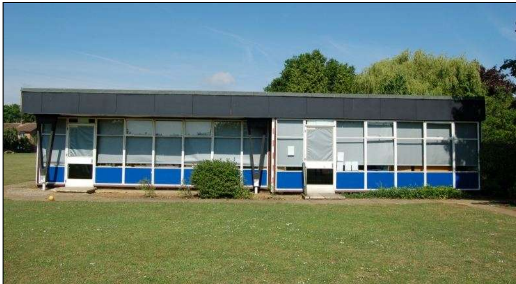
Plate 2: Block C, east elevation from east
