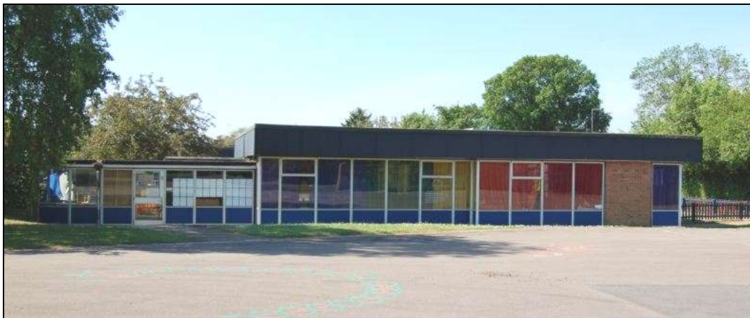
Plate 26: Block F and walkway, north elevation from north
