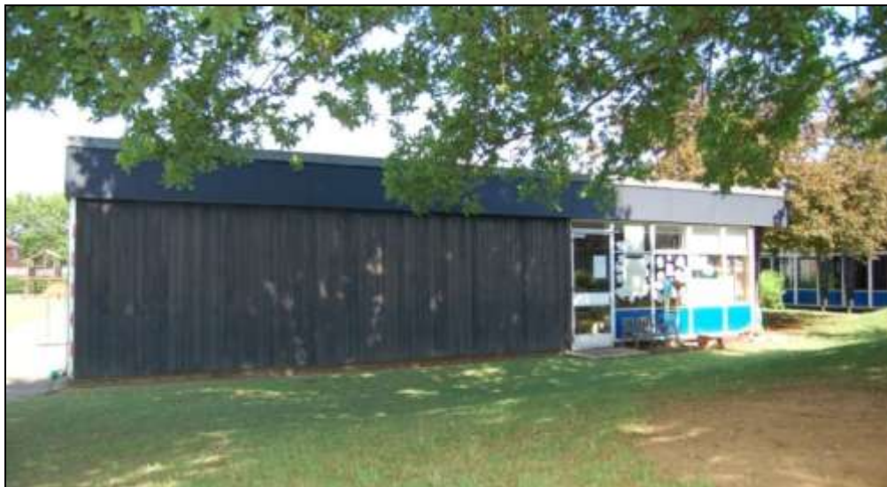
Plate 3: Block E, east elevation from east
