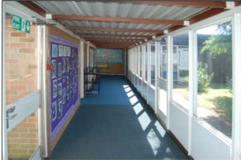
Plate 12: Walkway (174) between Blocks A & B, looking east
