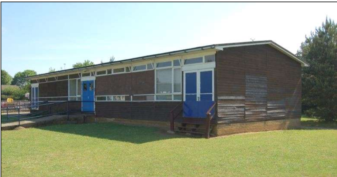
Plate 31: Block G, west elevation from south-west
