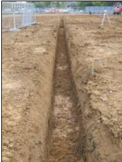
Plate 9: Footing trench in western part of site, looking east, 2m scale
