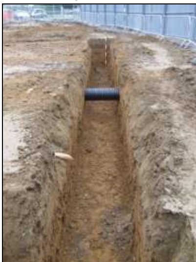
Plate 11: Footing trench in former car park, looking east, 2m scale
