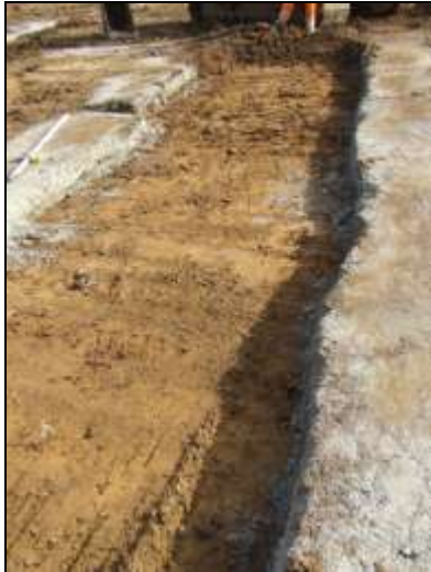
Plate 13: Ground reduction between footing trenches, looking north east
