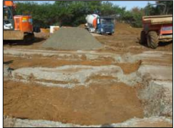
Plate 14: Ground reduction between footing trenches, showing evaluation trench, looking north
