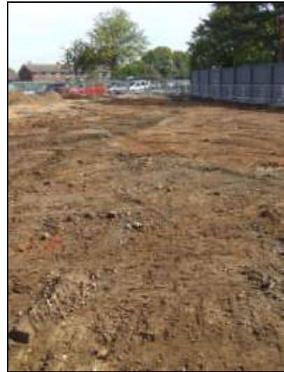
Plate 2: Car park after removal of tarmac, looking east
