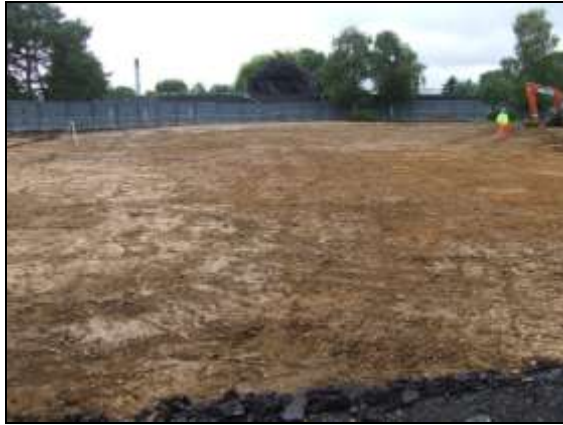
Plate 7: Site during levelling, looking south west
