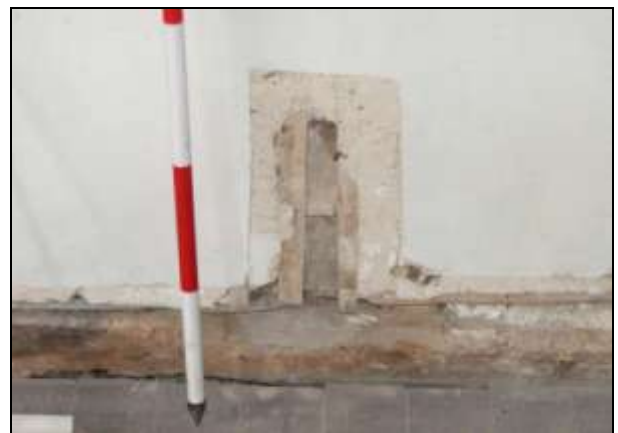
Plate 22: Room 4, north wall, weatherboarding beneath lath & plaster
