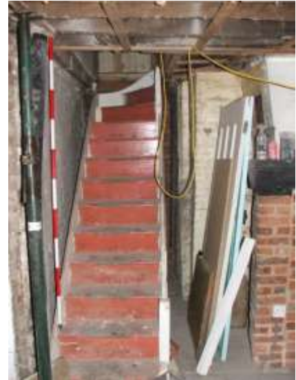
Plate 14: Room 1, stairs to first floor, looking south
