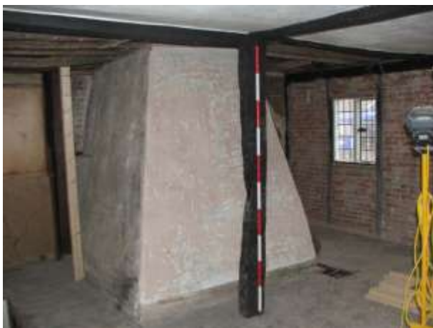
Plate 25: Room 4, chimney breast, view south-west
