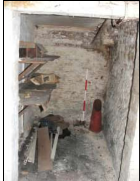
Plate 8: Cellar, northward extension beneath Room 3
