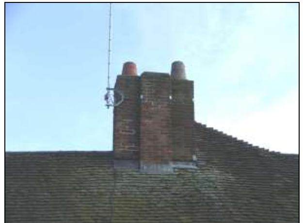
Plate 34: Chimney stack from west
