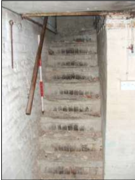
Plate 7: Cellar stairs, view north
