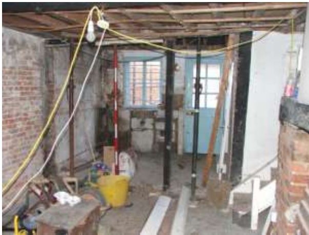
Plate 9: Room 1, general view east
