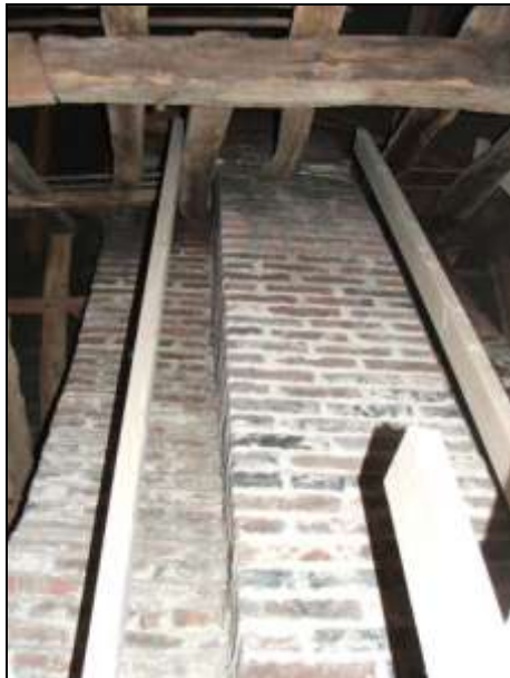
Plate 33: Roof space: chimney stack, east side
