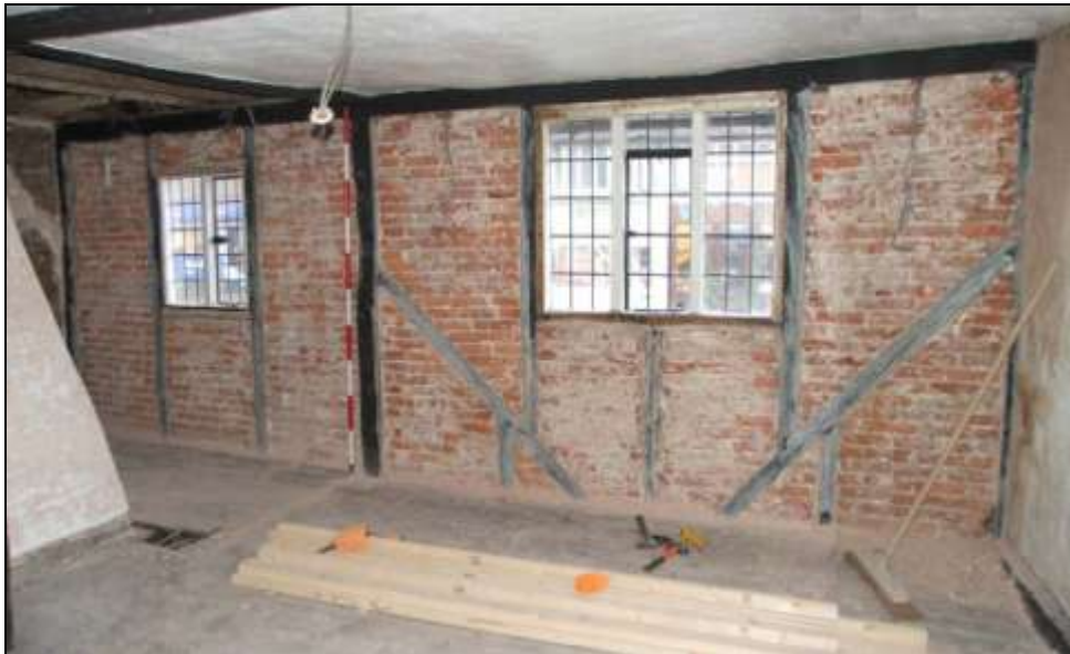
Plate 20: Room 4, west wall
