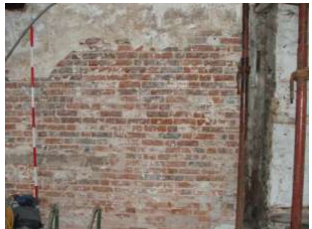
Plate 12: Room 1, north wall (east)
