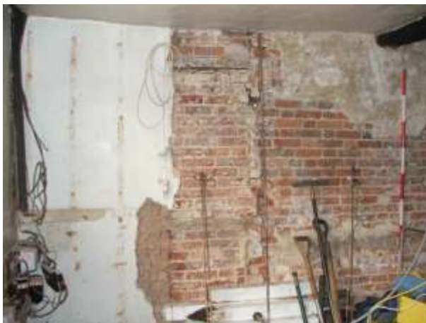
Plate 11: Room 1, north wall (west)
