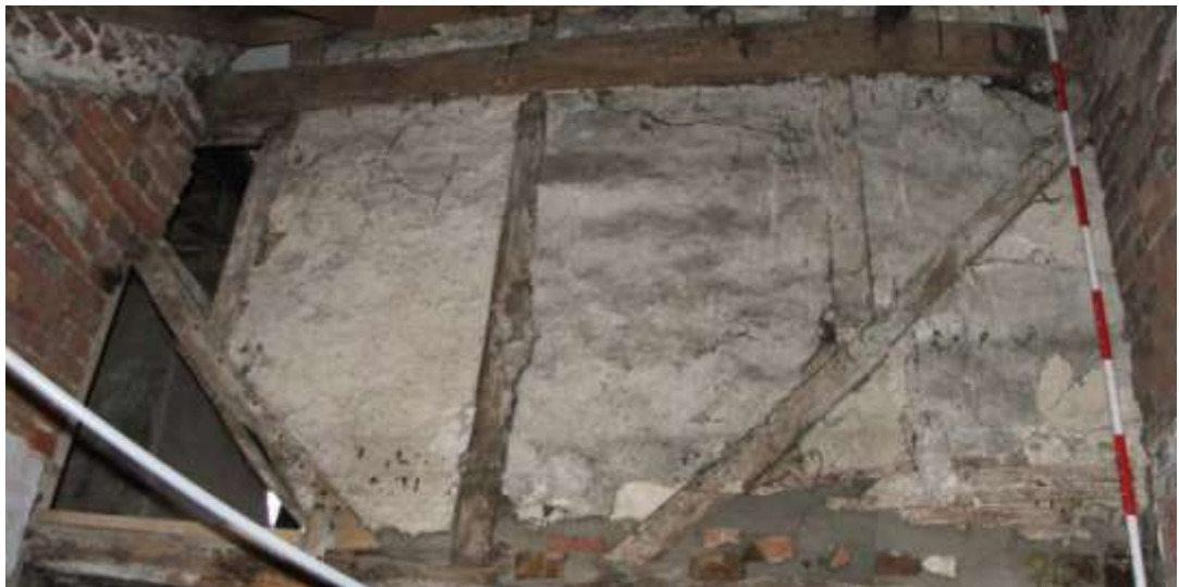
Plate 24: Original rear wall of building (opposite side of wall in Plate 23)
