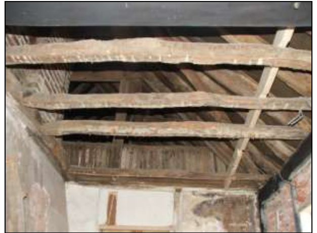
Plate 32: Room 4, ceiling joists, south-west corner
