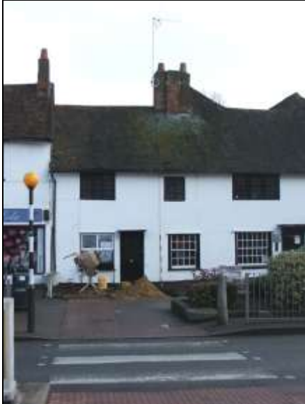
Plate 1: General view of building from west
