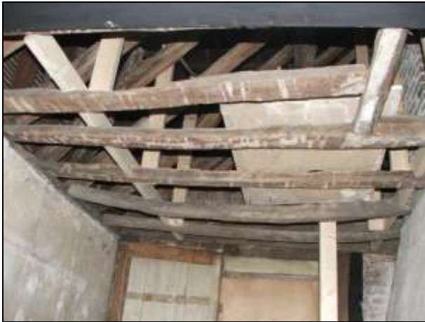
Plate 31: Room 4, ceiling joists, south-east corner
