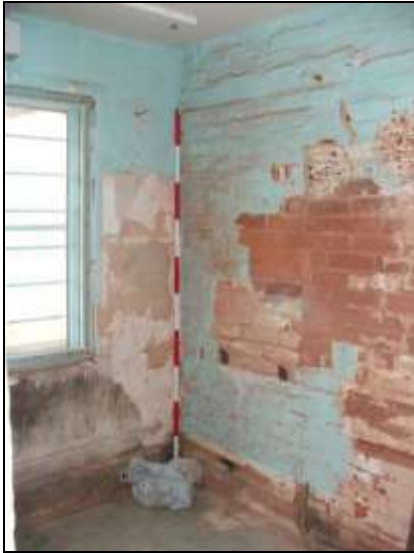
Plate 18: Room 3, view south-east
