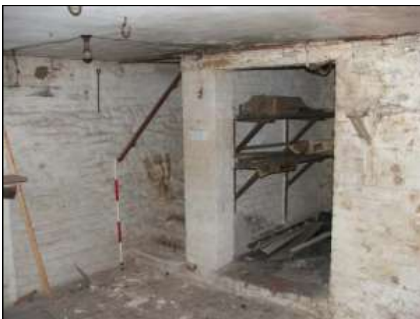
Plate 5: Cellar, view north-west
