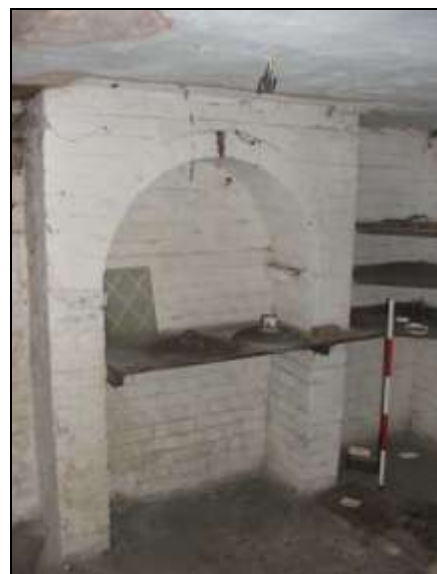
Plate 6: Cellar, view south-west
