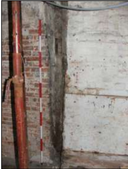
Plate 13: Room 1, jowled post in north wall
