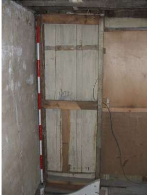
Plate 27: Room 4, south wall, panelling
