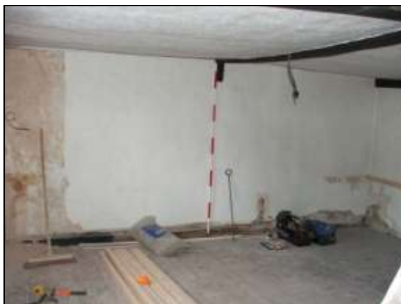
Plate 21: Room 4, north wall
