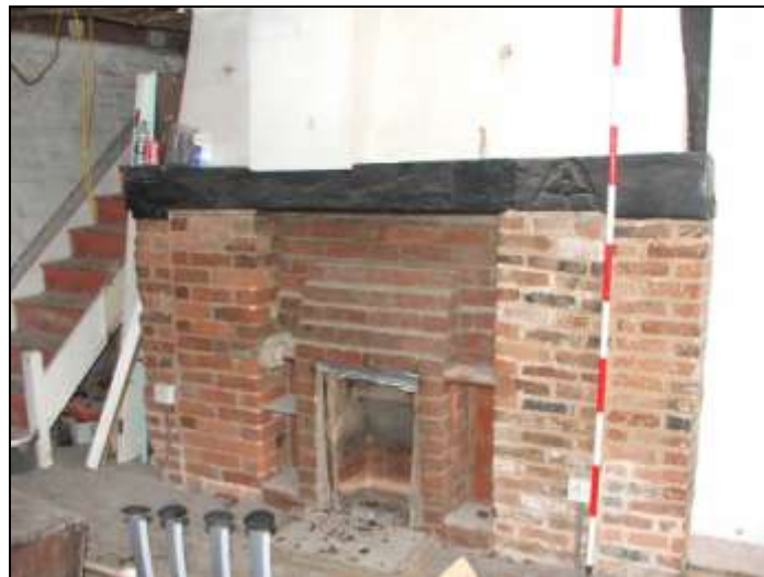
Plate 15: Room 1, fireplace looking south-east
