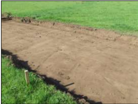
Plate 1: Driveway in the area of linear earthworks, looking southwest
