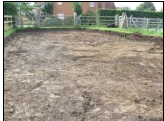
Plate 4: Areas of burning and rubble at southern end of driveway, looking south, 1m scale
