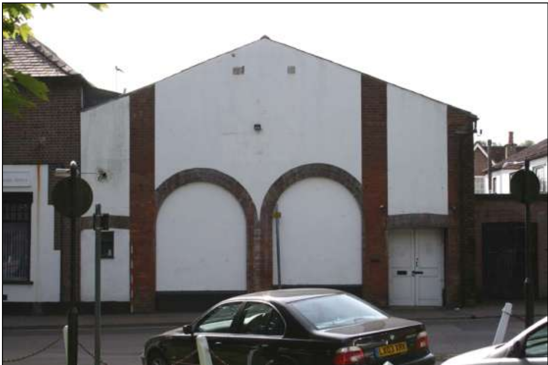
Plate 2: Victoria Works, north elevation
