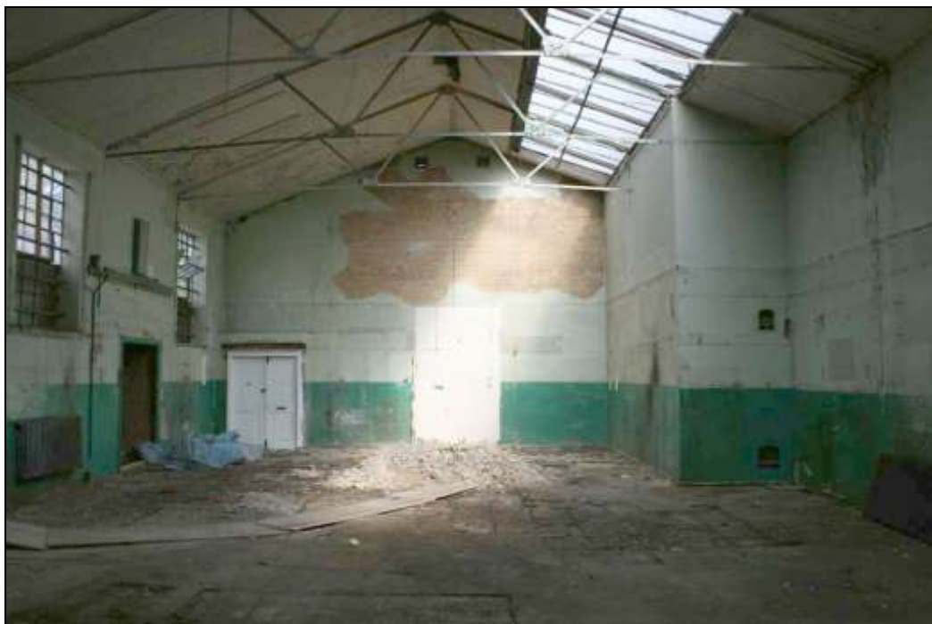
Plate 5: Victoria Works, G1 looking north
