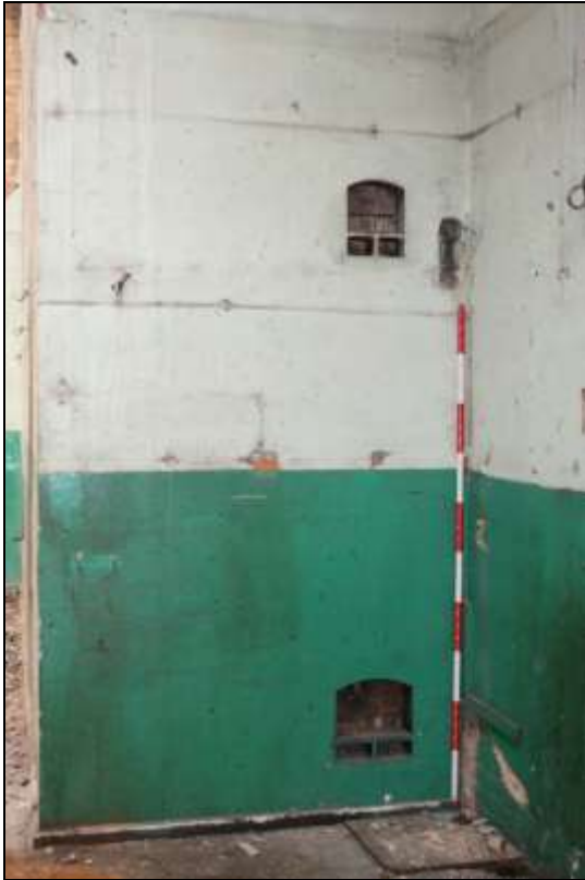
Plate 8: Victoria Works, G1, detail of bearing mounts in east wall
