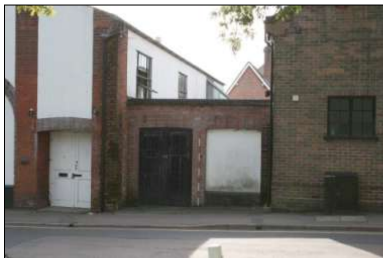
Plate 15: Link Building, north elevation
