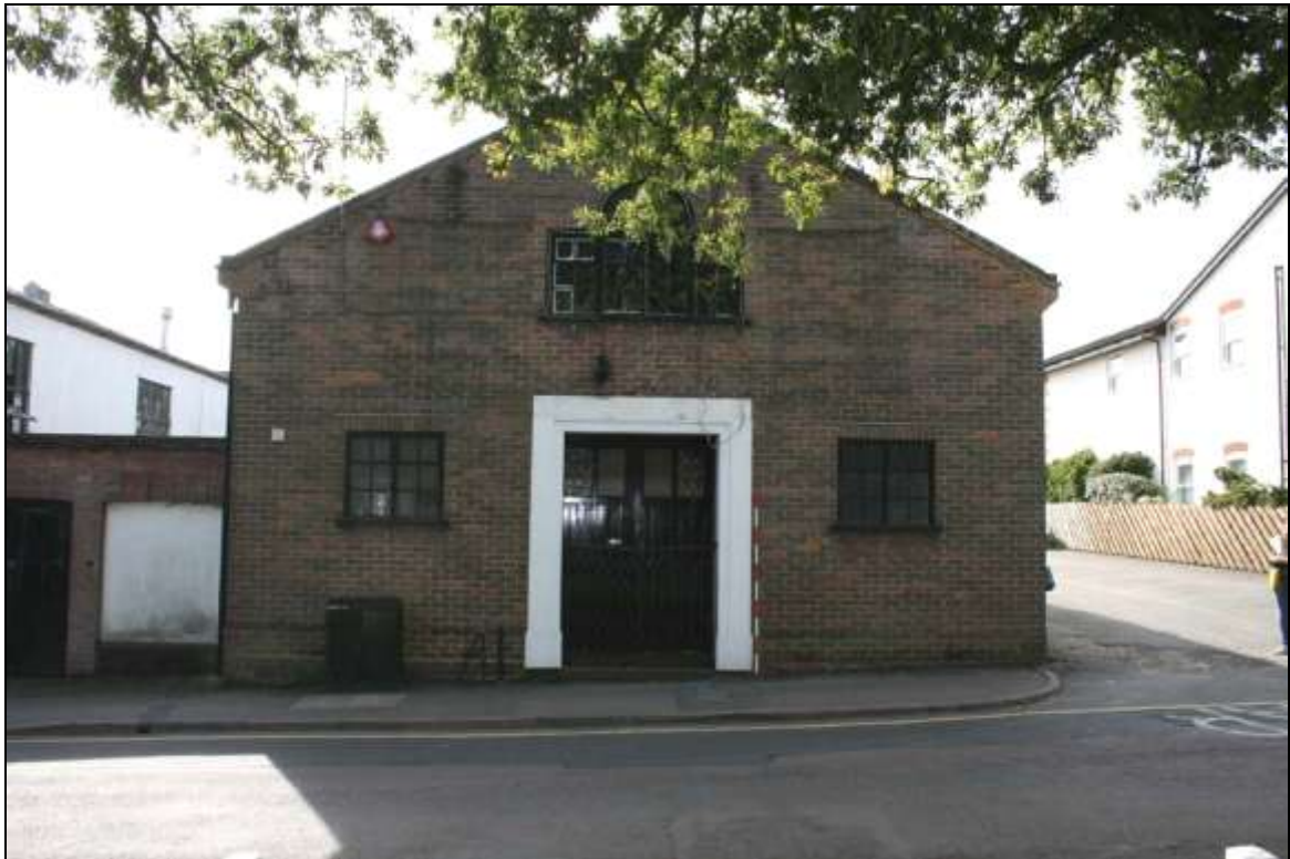
Plate 19: Leyton Hall, north elevation
