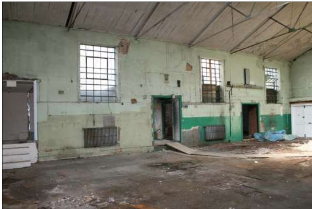
Plate 7: Victoria Works, G1 looking north-west
