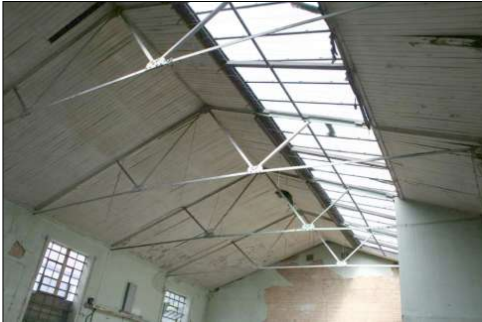
Plate 14: Victoria Works, roof structure
