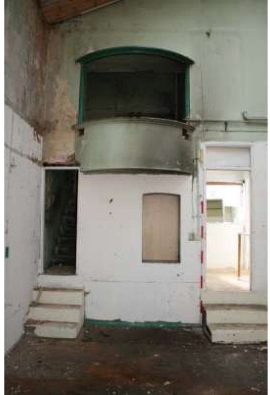
Plate 9: Victoria Works, G1, balcony and openings in south wall
