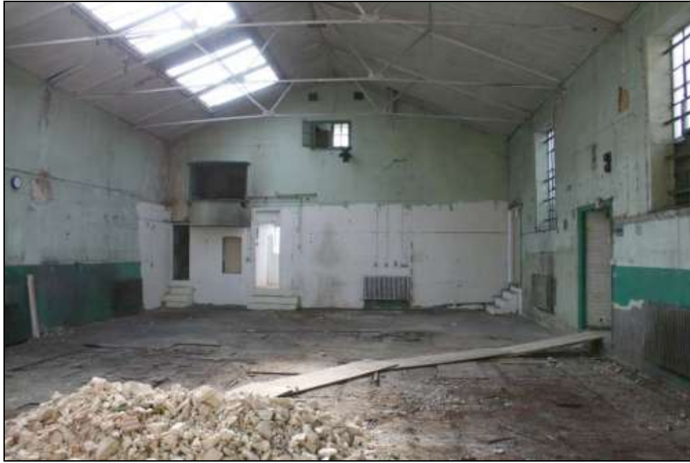
Plate 6: Victoria Works, G1 looking south
