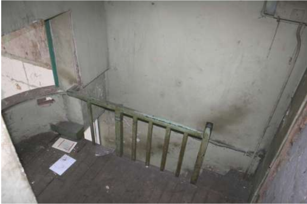
Plate 11: Victoria Works, F1 and stairwell
