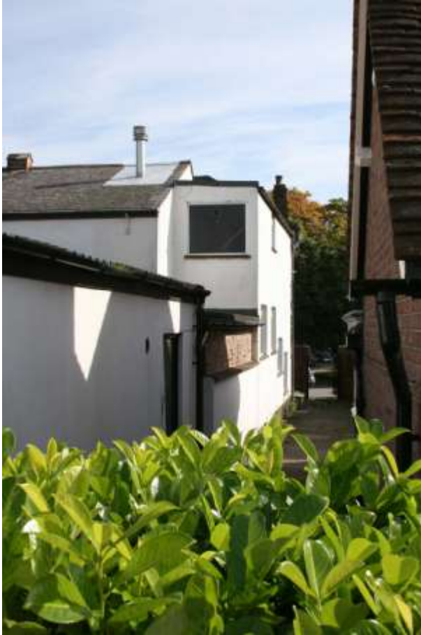
Plate 3: Victoria Works, south elevation from west
