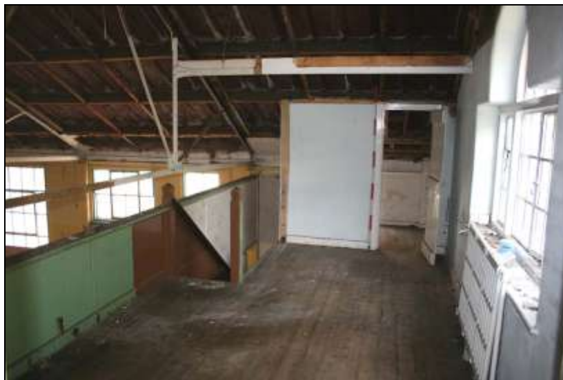
Plate 29: Leyton Hall, F3 & F4, looking west
