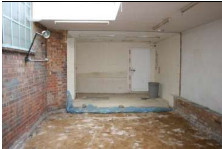
Plate 17: Link Building, G7 and G8, looking south
