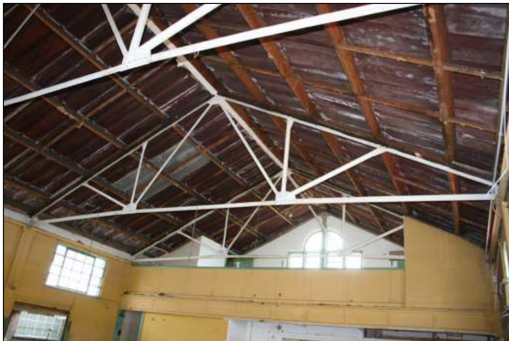
Plate 33: Leyton Hall, roof structure
