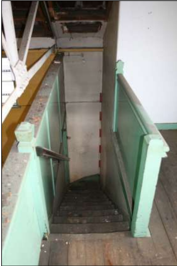
Plate 31: Leyton Hall, F6, stairway
