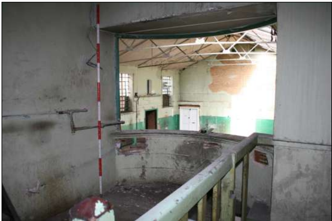
Plate 10: Victoria Works, F1, looking north
