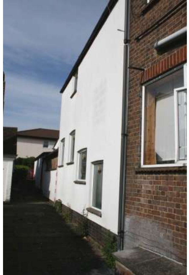
Plate 4: Victoria Works, south elevation from east
