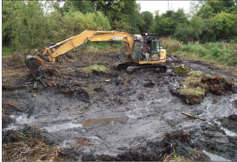
Plate 1: The pond under excavation
