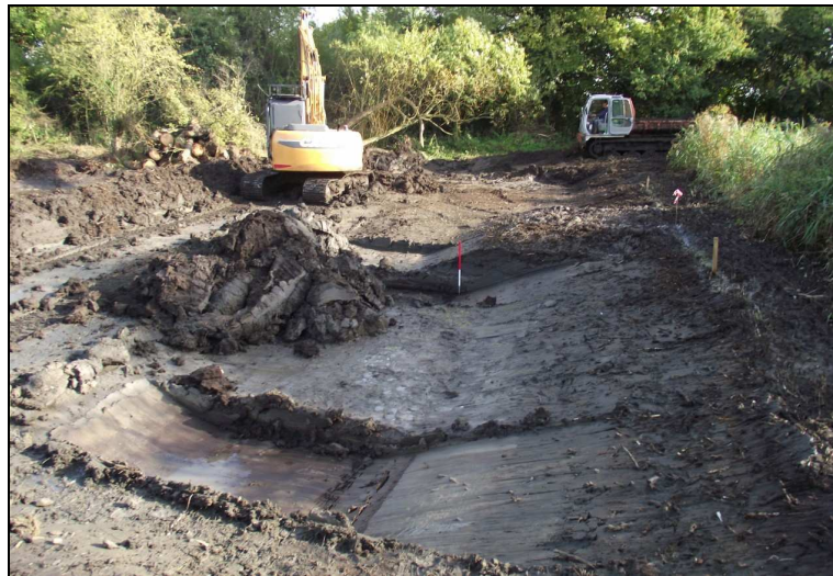
Plate 2: The pond under excavation
