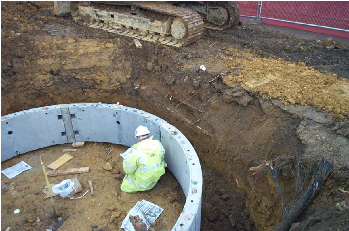
Plate 1: Area 1 excavation, looking north east
