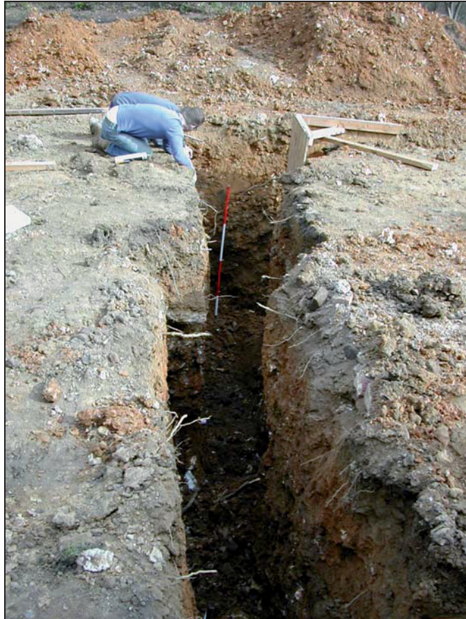
Plate 1: A typical section of footing trench
