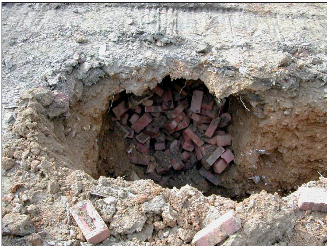
Plate 2: Mid 20 th century Soakaway filled with Fletton bricks
