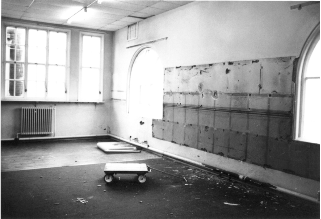
Plate 24: Rooms 4 & 5, c.1980, looking north west
