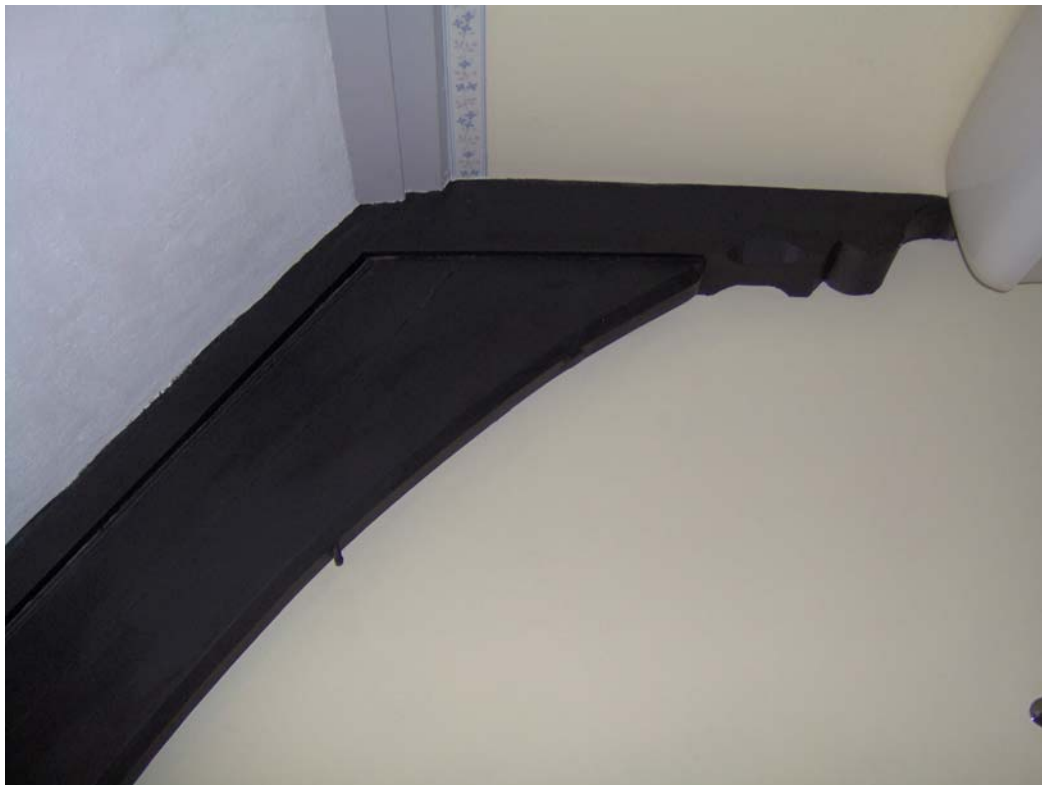
Plate 21: Room 16, detail of roof truss, south wall
