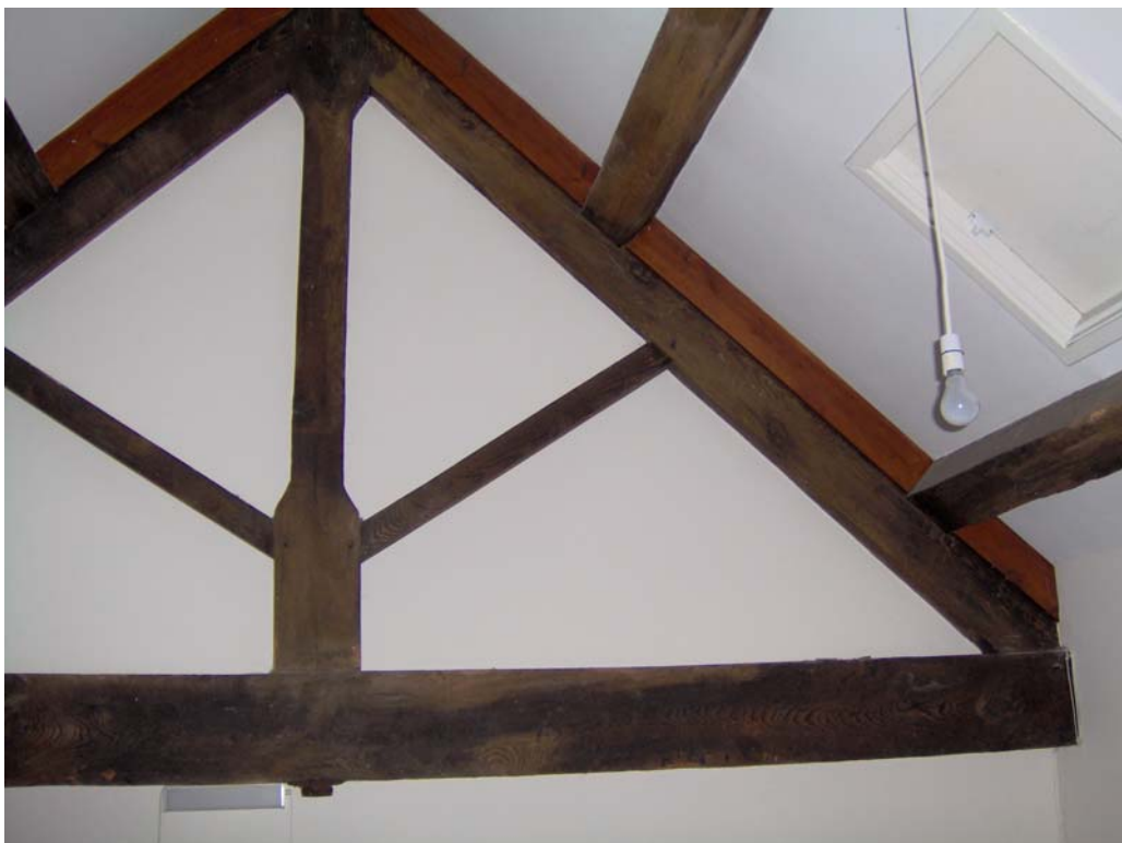
Plate 19: Room 14, detail of roof truss
