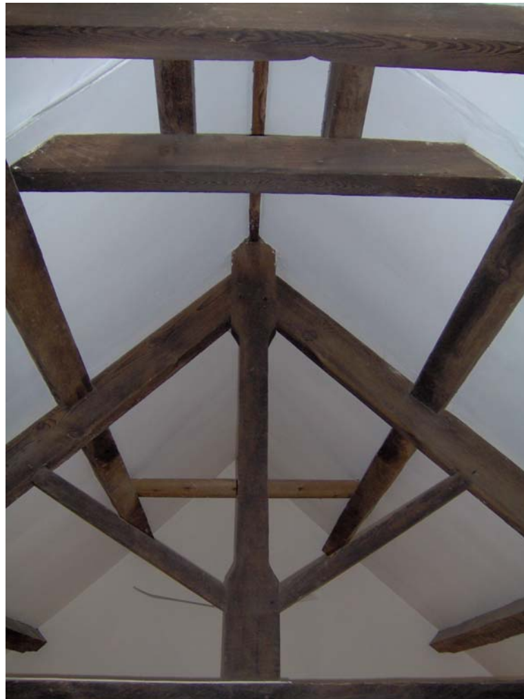
Plate 12: Room 5, detail of roof truss
