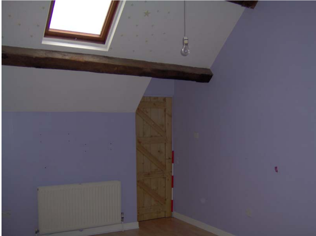
Plate 20: Room 15, looking south west
