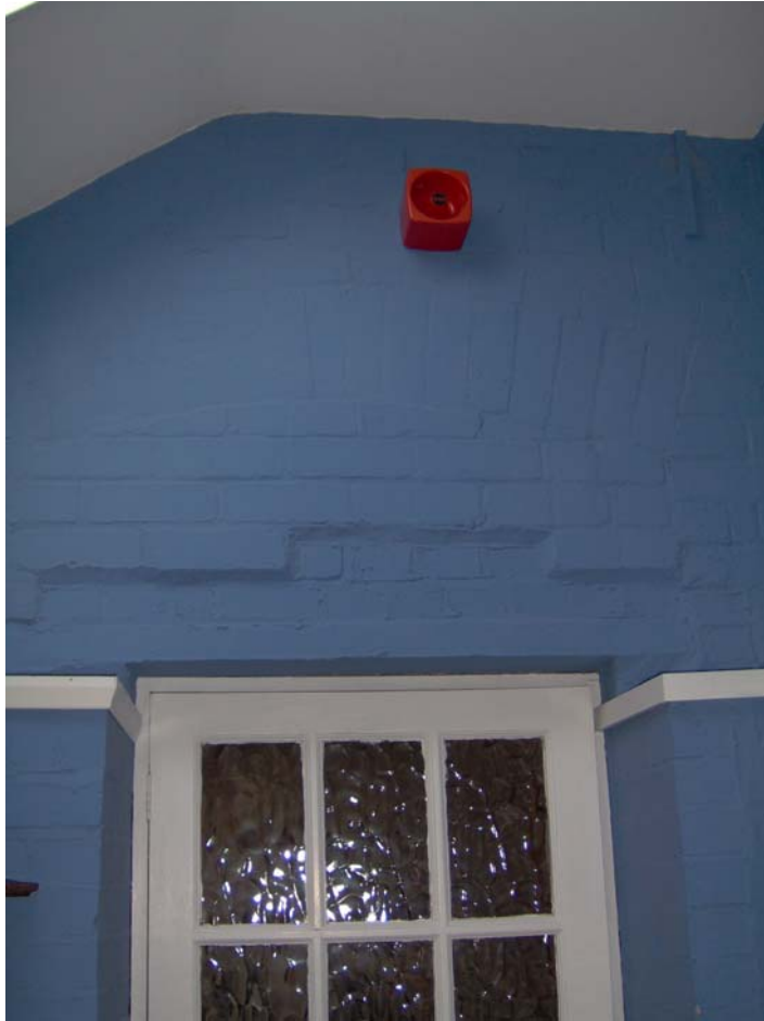
Plate 16: Room 9, detail of bricked up entrance on north wall
