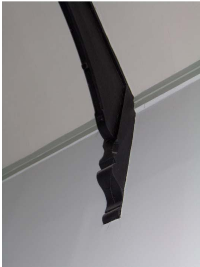
Plate 15: Room 7, roof truss detail
