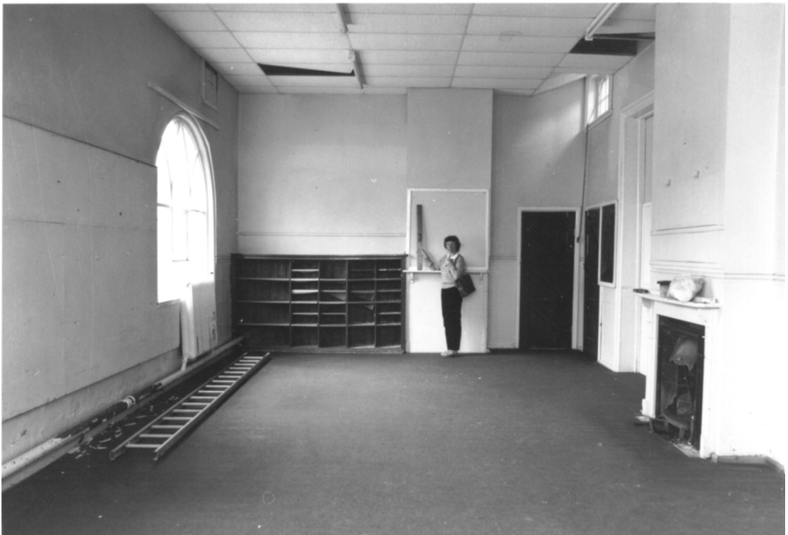
Plate 25: Rooms 4 & 5, c.1980, looking east
