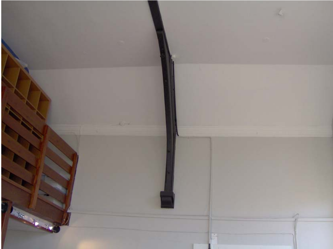
Plate 8: Room 2, detail of roof truss
