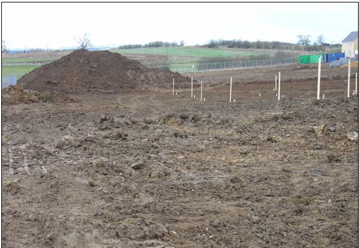
Plate 6. Site 3B showing topsoil store and site cabins, looking west
