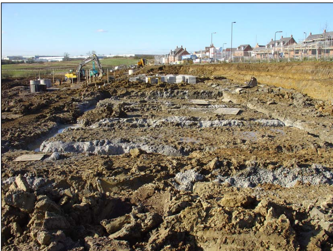
Plate 4. Site 3A; footings in northern terrace, looking west
