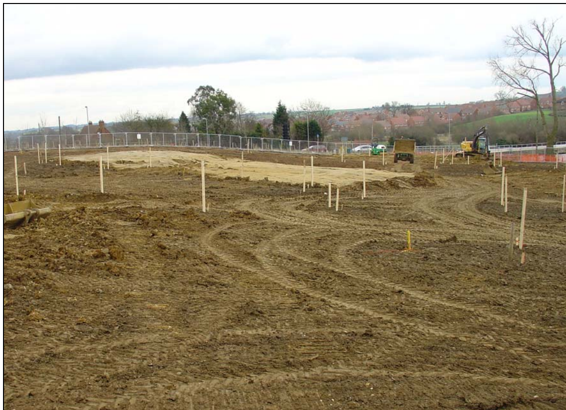
Plate 8. Site 3C; deposition of levelling material, looking east
