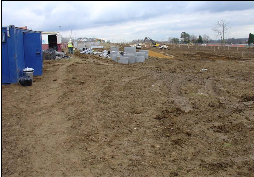
Plate 1. General site shot during topsoil strip, looking east
