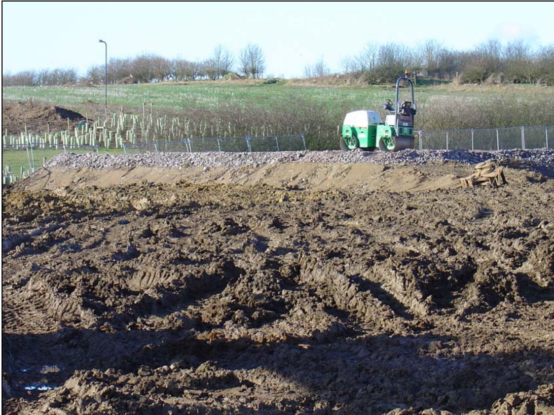
Plate 7. Site 3B; deposition of levelling material, looking southwest
