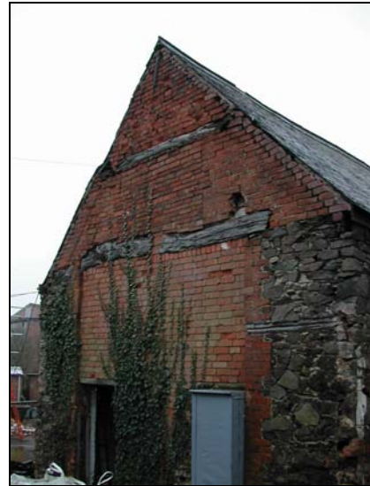
Plate 8: Building 1, west end
