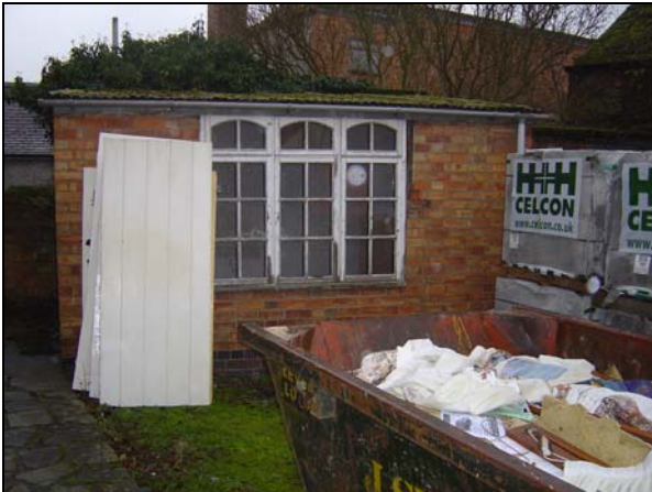
Plate 27: Building 3, south elevation
