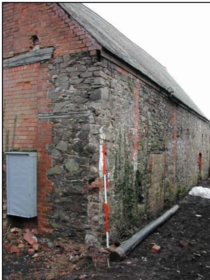
Plate 9: Building 1, south-west corner
