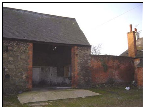
Plate 12: Building 1, cart door in north elevation
