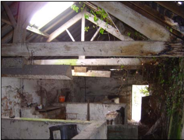
Plate 25: Building 2, roof structure
