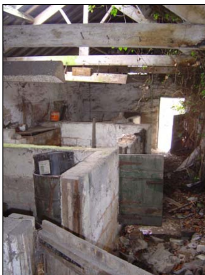
Plate 23: Building 2 interior, looking south
