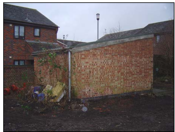
Plate 30: Building 4, from north-east
