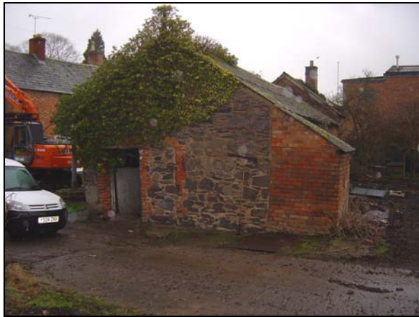
Plate 21: Building 2, south elevation
