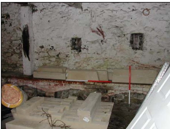
Plate 17: Building 1, brick bench in east central bay
