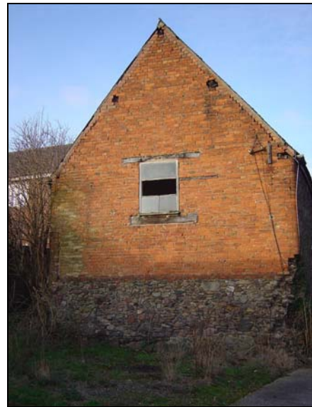
Plate 10: Building 1, east end
