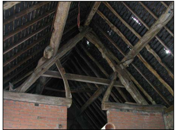
Plate 14: Building 1, roof structure looking east
