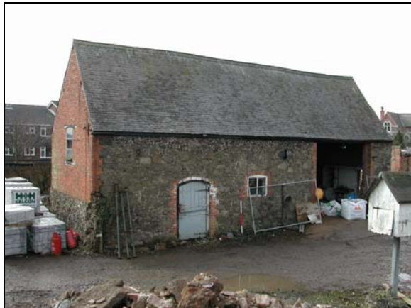
Plate 7: Building 1, north elevation.
