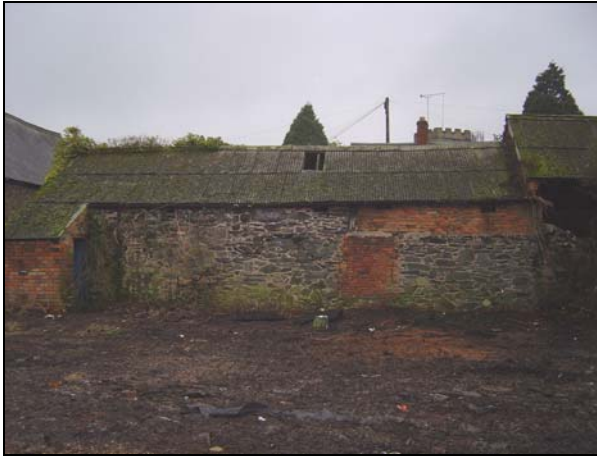
Plate 19: Building 2, east elevation
