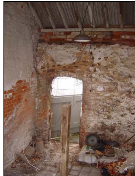
Plate 26: Building 2, inside north end
