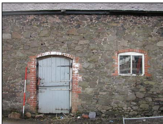
Plate 11: Building 1, stable door in north elevation
