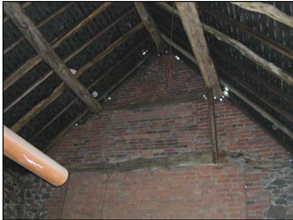
Plate 15: Building 1, roof structure looking west
