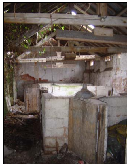
Plate 24: Building 2 interior, looking north
