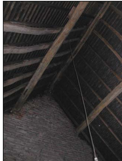
Plate 16: Building 1, east gable end
