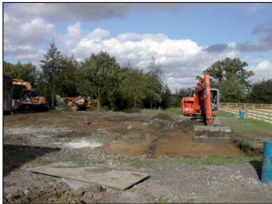
Plate 3: Ground reduction underway
