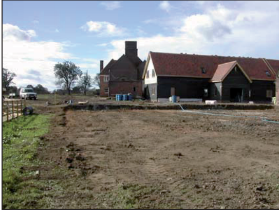
Plate 7: Completed ground reduction
