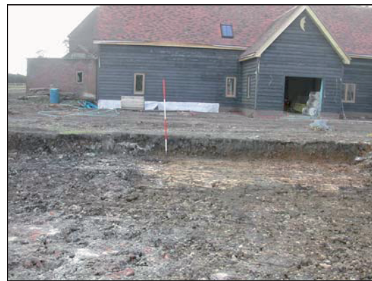
Plate 6: Detail of ground make-up of south section
