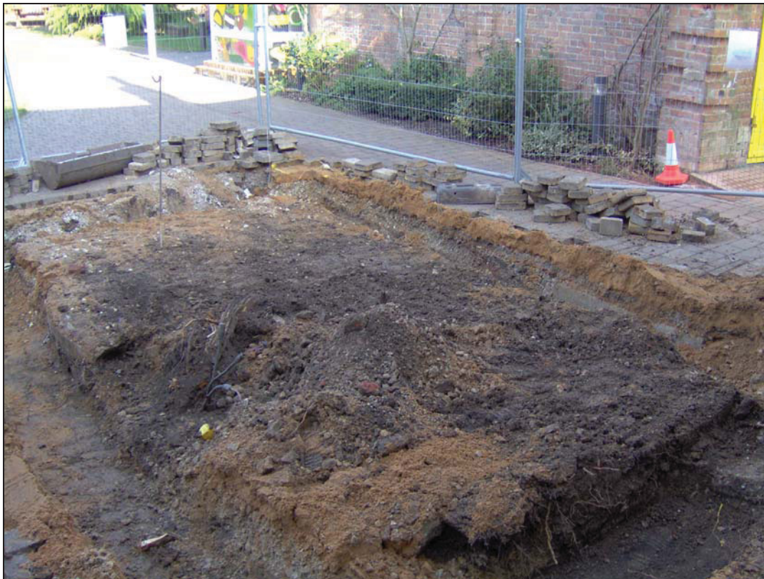
Plate 2: Completed Foundation Trench, looking East
