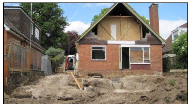
Plate 6: General view of site with completed footings looking north.
