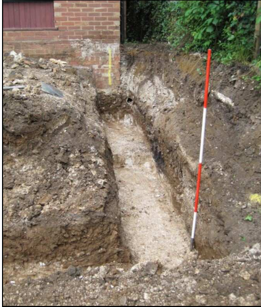
Plate 1: South east footings looking north
