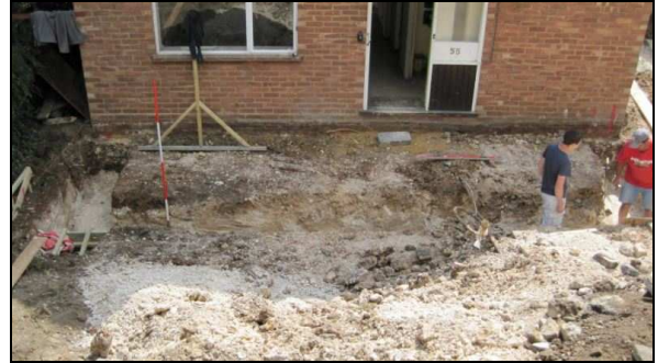
Plate 2: Foundation trenches in front of house
