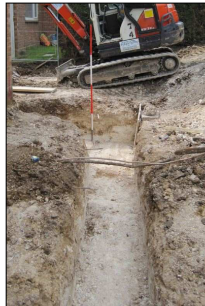
Plate 4: Foundation trench looking west
