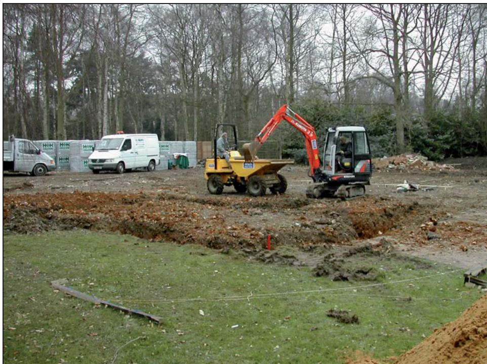
Plate 2: General view of the site during excavations
