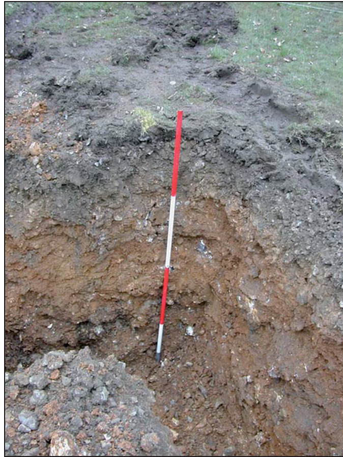
Plate 1: A typical section of the footing trench
