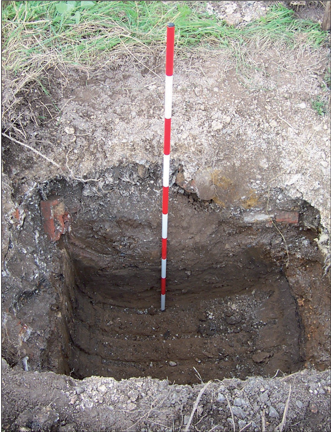
Plate 3: Foundation Pit 1 (looking northwest)
