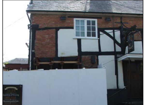
Plate 2: Lowndes Arms: area undergoing repairs
