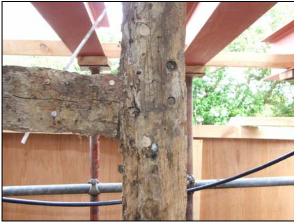
Plate 7: Timbers C & E junction, internal view
