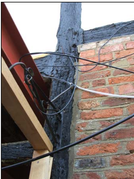
Plate 5: Timber D, junction with F
