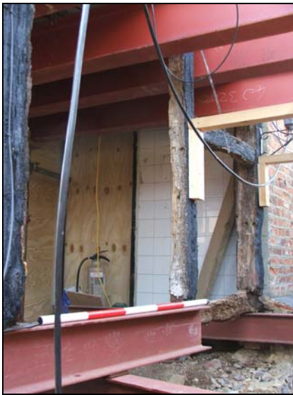
Plate 3: Repair area, view from north-west
