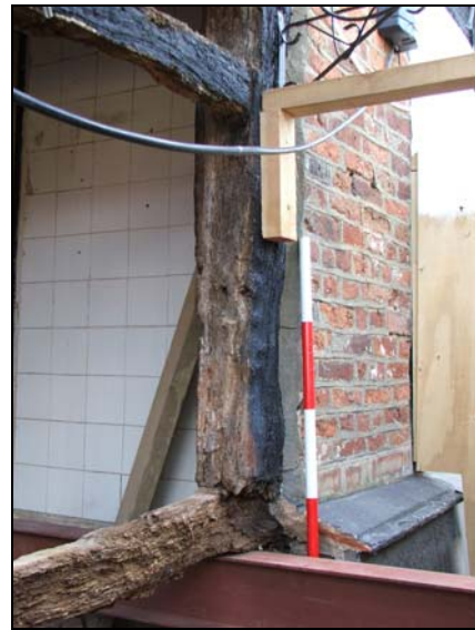
Plate 4: Timbers A, D & E, from north-west
