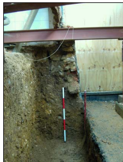
Plate 12: Section revealed by removal of wall
