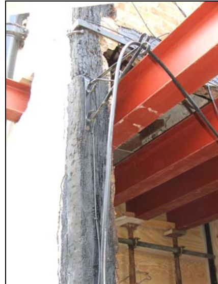
Plate 8: Timber B, junction with F
