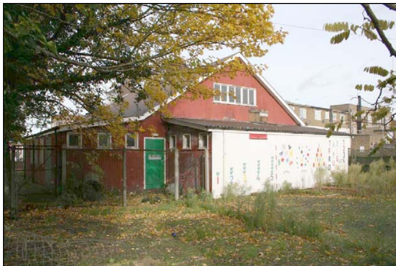
Plate 3: Church Hall: south-east elevation, from south
