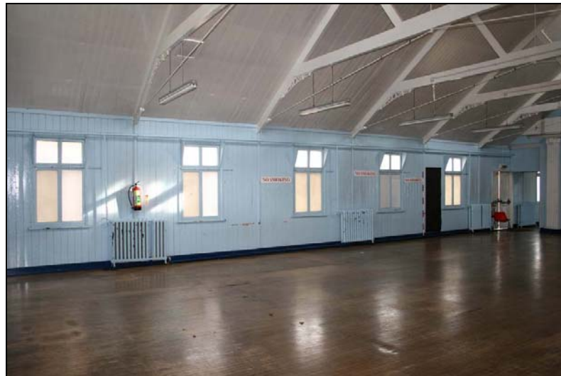
Plate 7: Church Hall: hall interior, looking east
