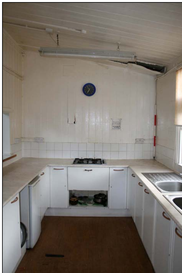
Plate 17: Church Hall: kitchen, looking south-east
