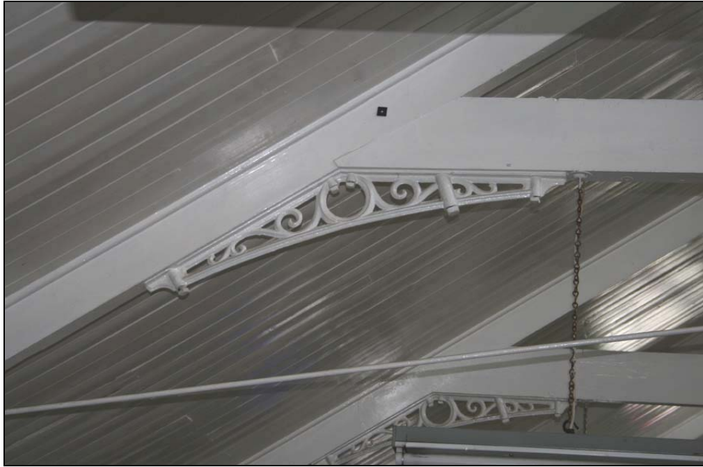
Plate 10: Church Hall: close-up of cast iron bracket on roof truss
