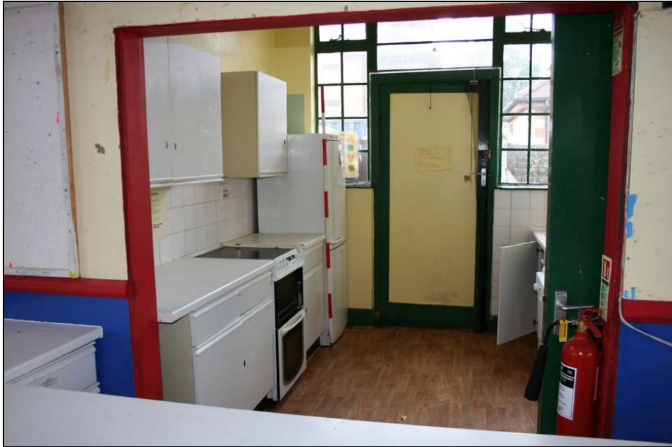
Plate 33: Nursery: Room G8 kitchen, looking south-west
