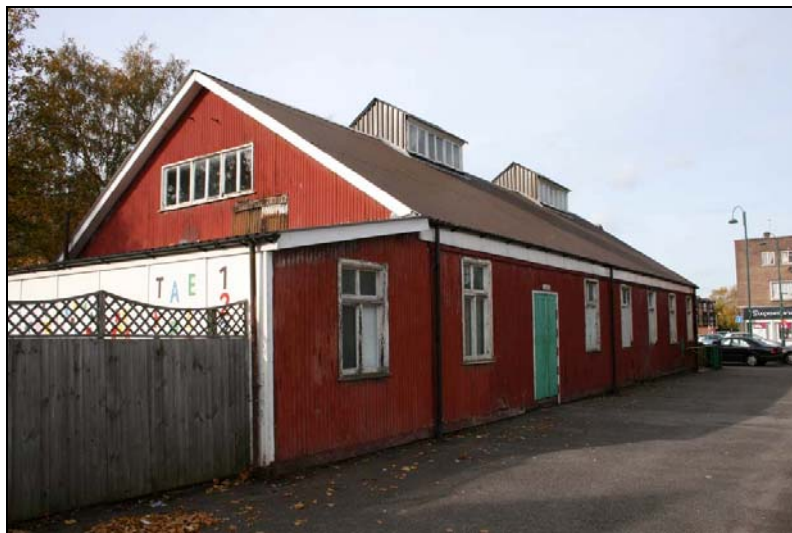
Plate 2: Church Hall: north-east elevation from east
