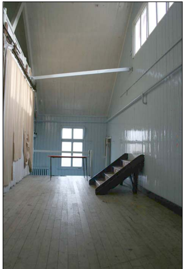
Plate 12: Church Hall: stage area looking north-east
