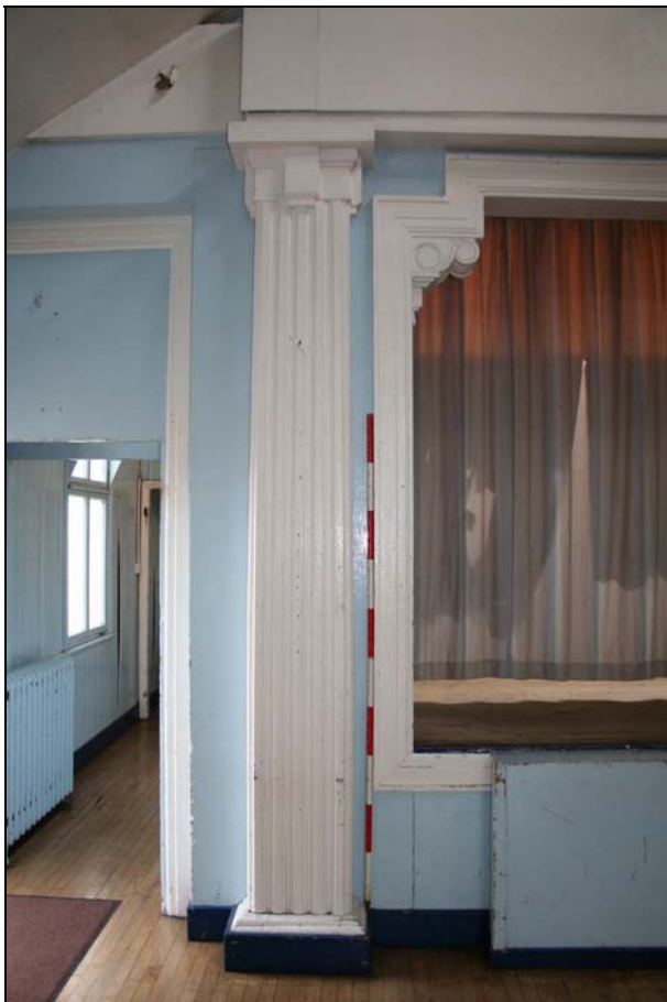
Plate 11: Church Hall: hall, detail of proscenium arch
