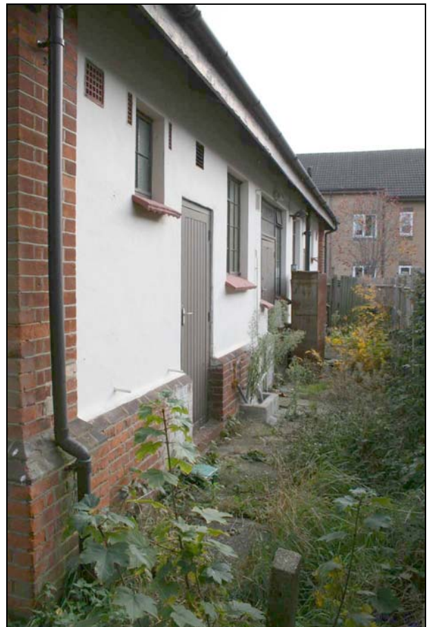
Plate 23: Nursery: south-west elevation, from north-west
