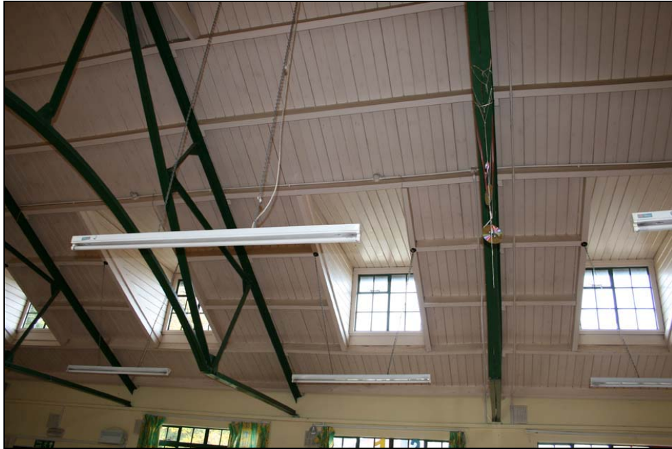
Plate 30: Nursery: Room G6, hall, detail of roof construction
