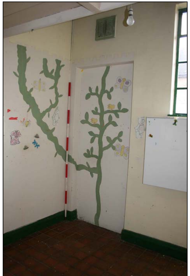
Plate 32: Nursery: Room G9, blocked doorway looking south
