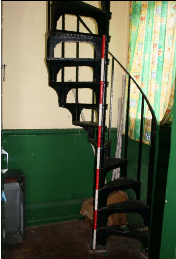
Plate 24: Nursery: Room G2, spiral stairs, looking north
