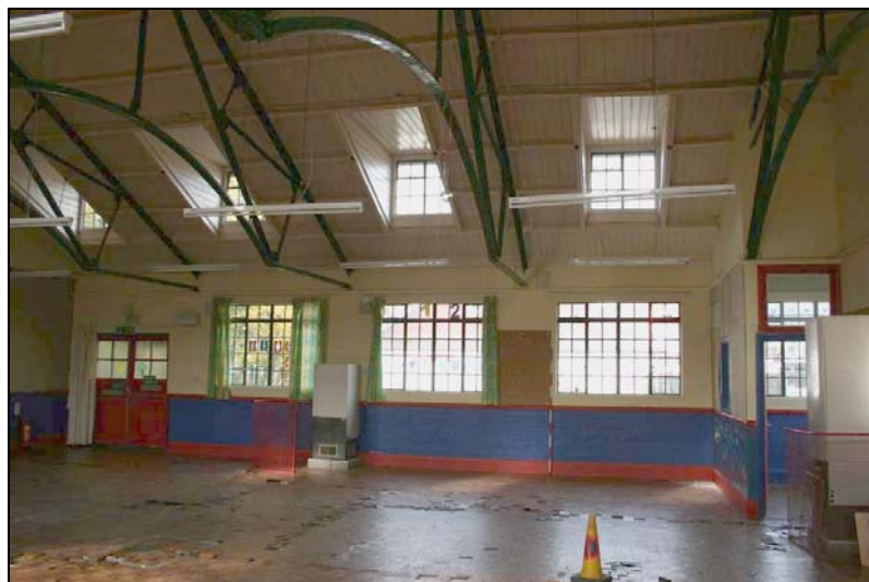
Plate 29: Nursery: Room G6, hall, looking north-west
