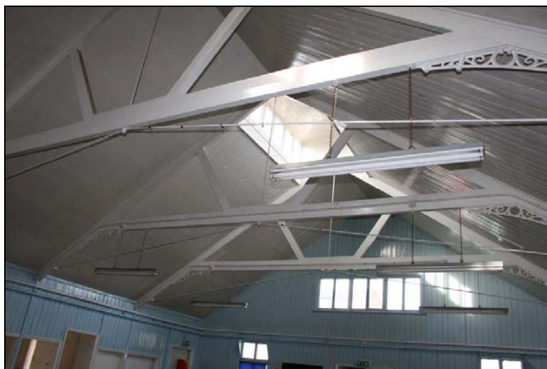
Plate 9: Church Hall: hall interior, detail of roof construction
