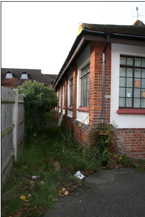
Plate 22: Nursery: south-east elevation, from north-east
