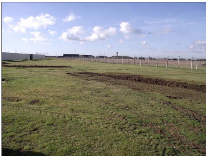
Plate 3: Backfilled trenches, looking west
