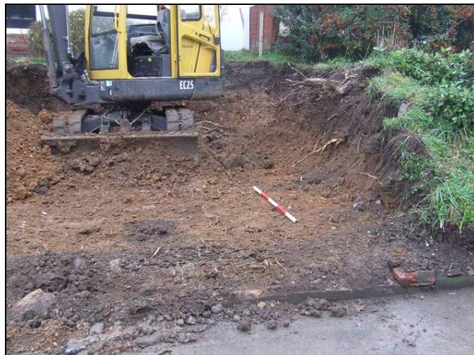
Plate 3: Ground reduction, looking north, 1m scale
