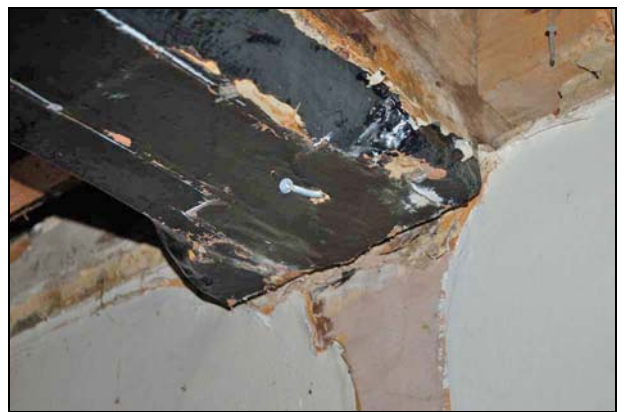
Plate 48: Lamb's tongue chamfer stop (Room G4)
