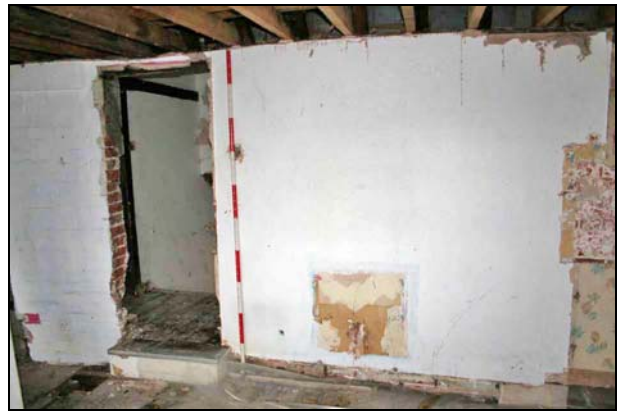
Plate 32: Room F6: west wall
