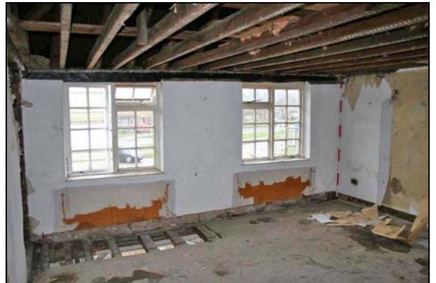
Plate 34: Room F7: east wall
