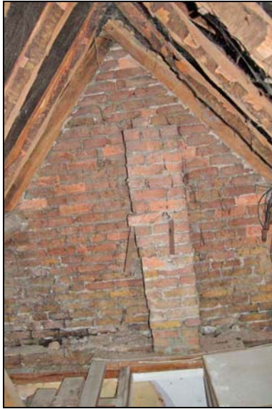
Plate 43: F7 roof: looking south
