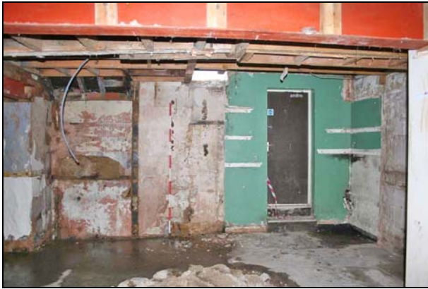
Plate 13: Room G4: west wall
