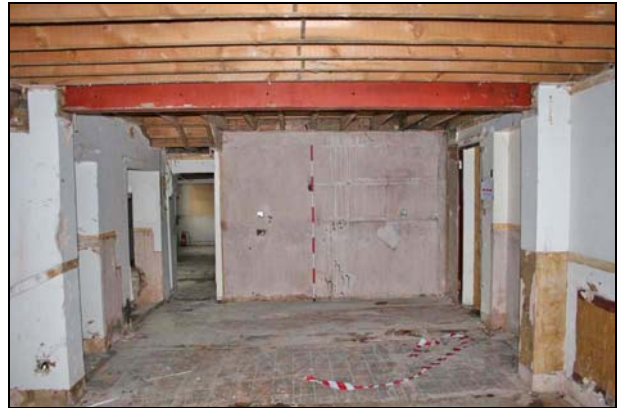
Plate 8: Room G1: south wall
