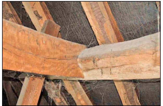
Plate 44: F7 roof: collar/purlin detail
