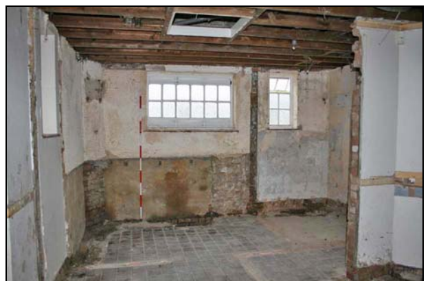
Plate 18: Room G6: west wall
