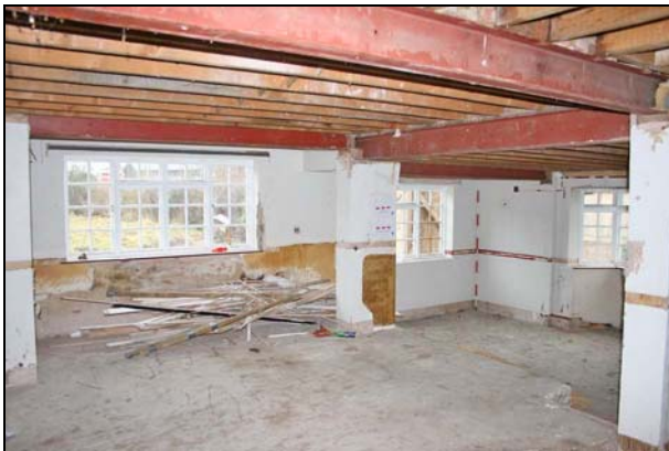
Plate 9: Rooms G1 & G2: north wall
