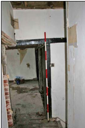
Plate 23: Room F2: looking south
