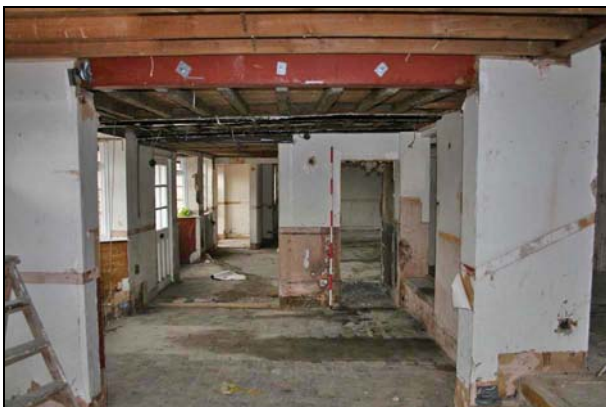
Plate 11: Rooms G2 & G3: looking south
