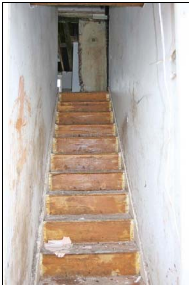
Plate 21: Room F1: Staircase
