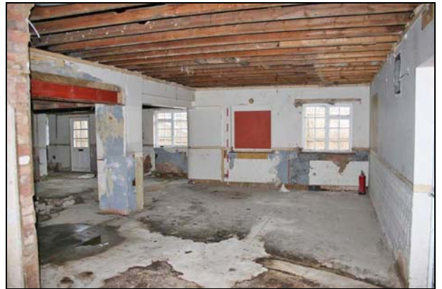
Plate 16: Room G5: east wall
