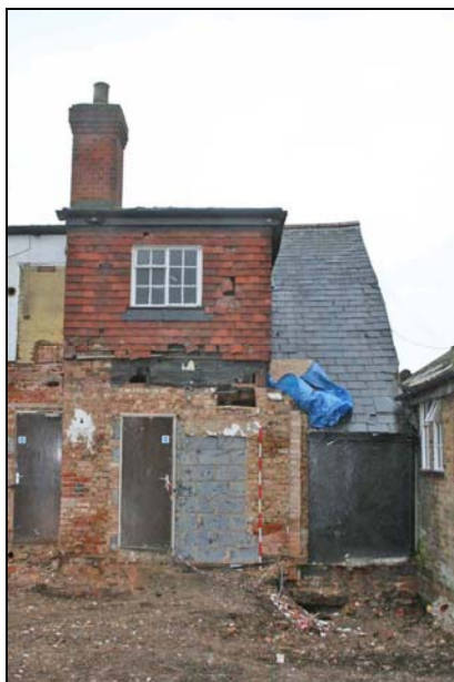
Plate 5: South end of west elevation
