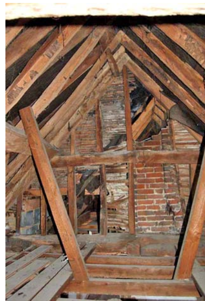
Plate 42: F7 roof: looking north
