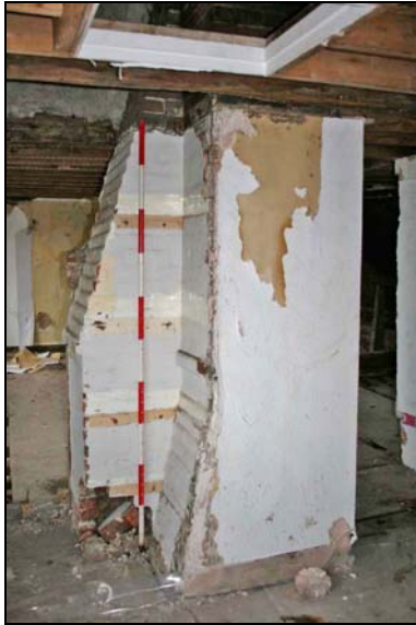
Plate 31: Room F6: chimney breast
