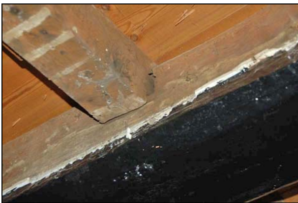
Plate 47: Ceiling joist detail (Room G3)
