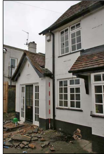
Plate 2: Southern end of east elevation
