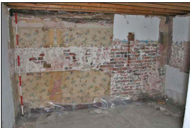
Plate 29: Room F6: north wall
