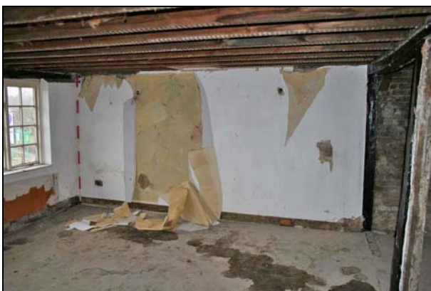
Plate 35: Room F7: south wall
