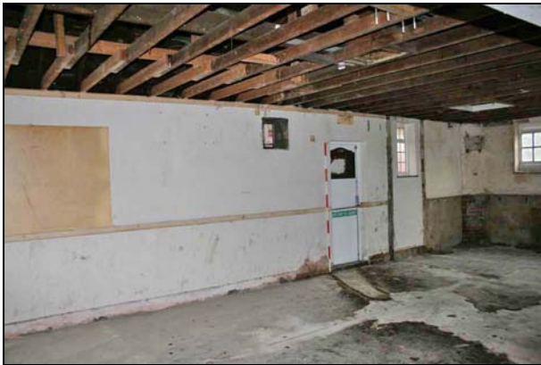
Plate 15: Room G5: south wall
