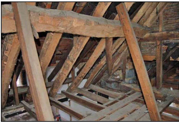
Plate 45: F7 roof: west side
