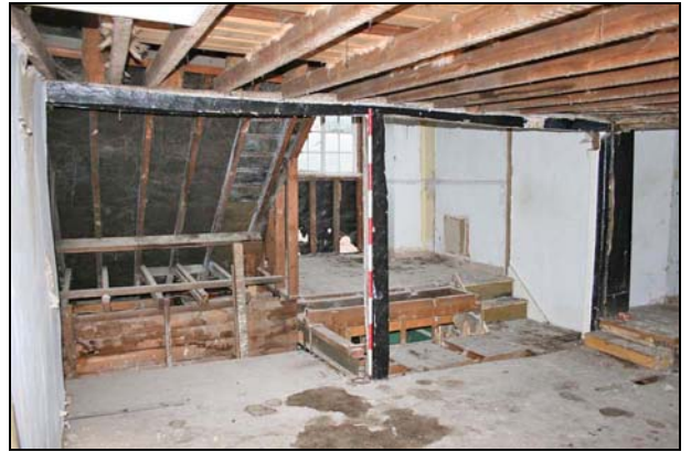
Plate 38: Room F7: looking northwest
