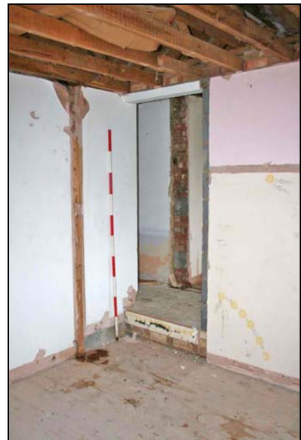
Plate 28: Room F5: southwest corner
