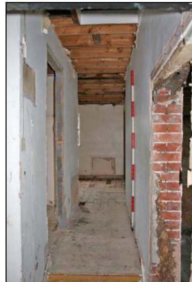
Plate 22: Room F2: looking north
