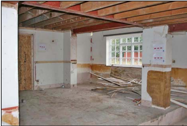
Plate 7: Room G1: northwest corner
