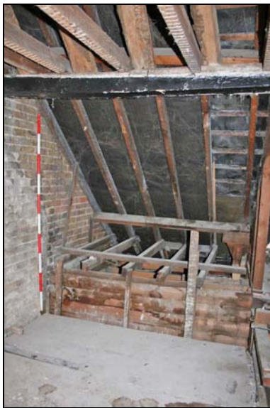
Plate 39: Room F7: catslide roof
