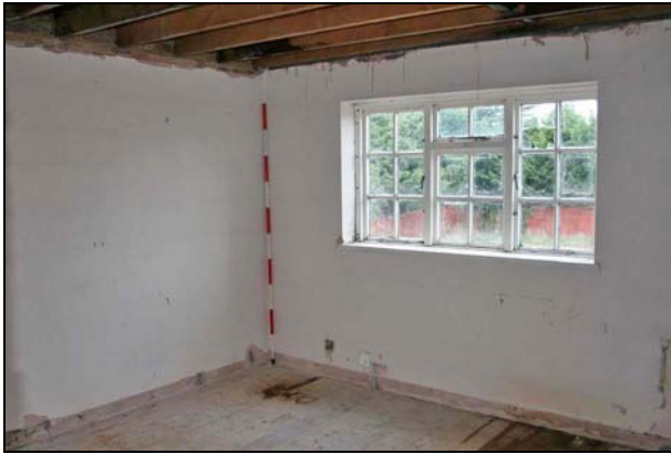
Plate 25: Room F4: northwest corner
