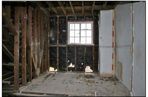
Plate 40: Room F8: looking east
