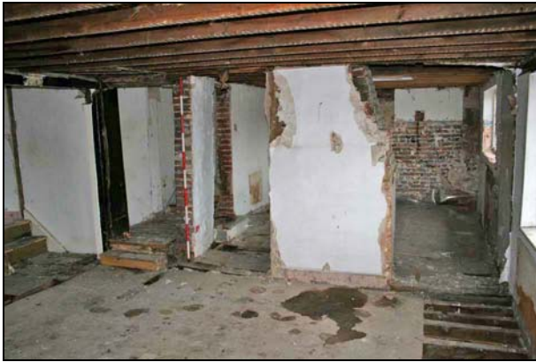
Plate 37: Room F7: north wall
