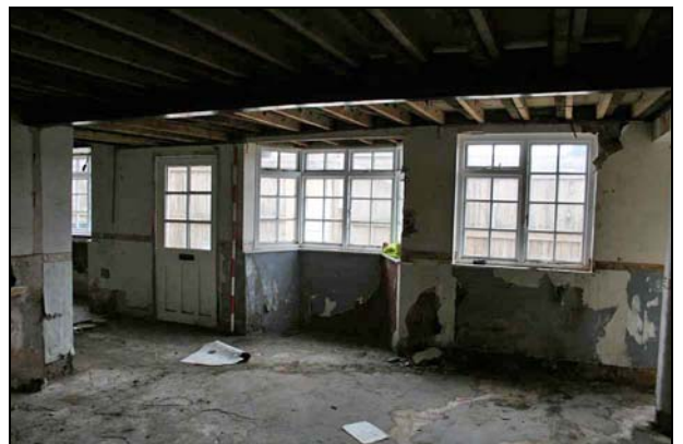
Plate 12: Room G4: east wall
