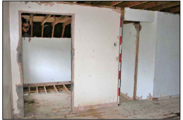
Plate 26: Room F4: looking southeast
