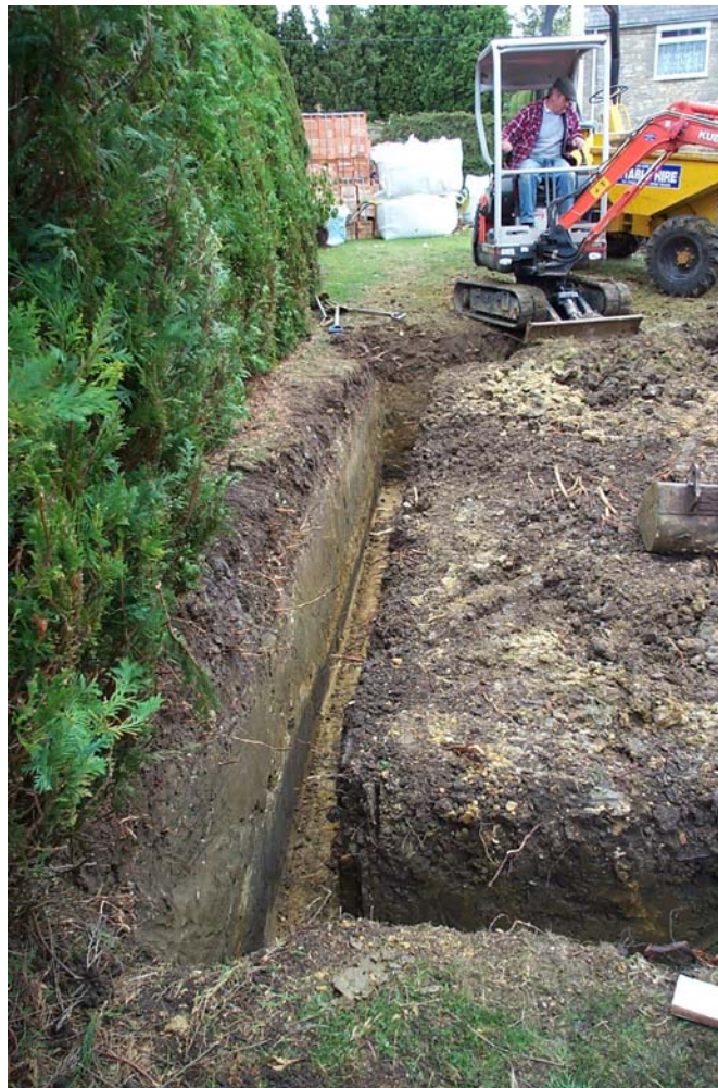
Plate 1: View of the garage footing trench
