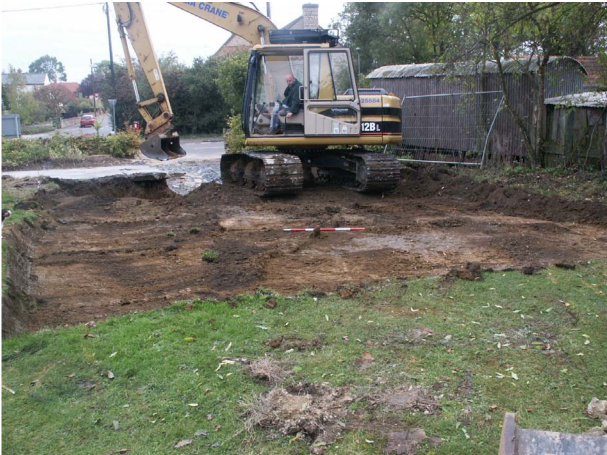
Plate 1: View of the site after the removal of the topsoil
