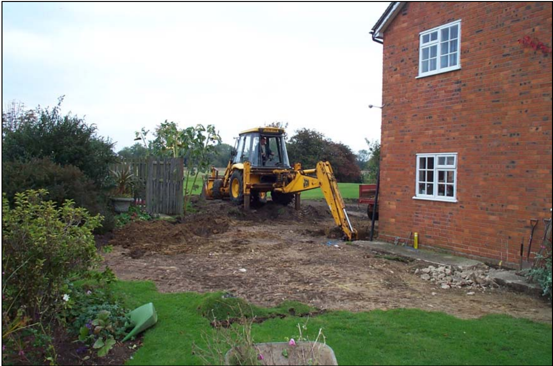
Plate 1: Excavation of the Foundations in Progress, looking East
