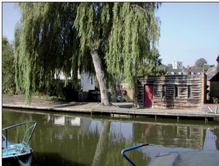
Plate 8: Garage & wharf, looking SW
