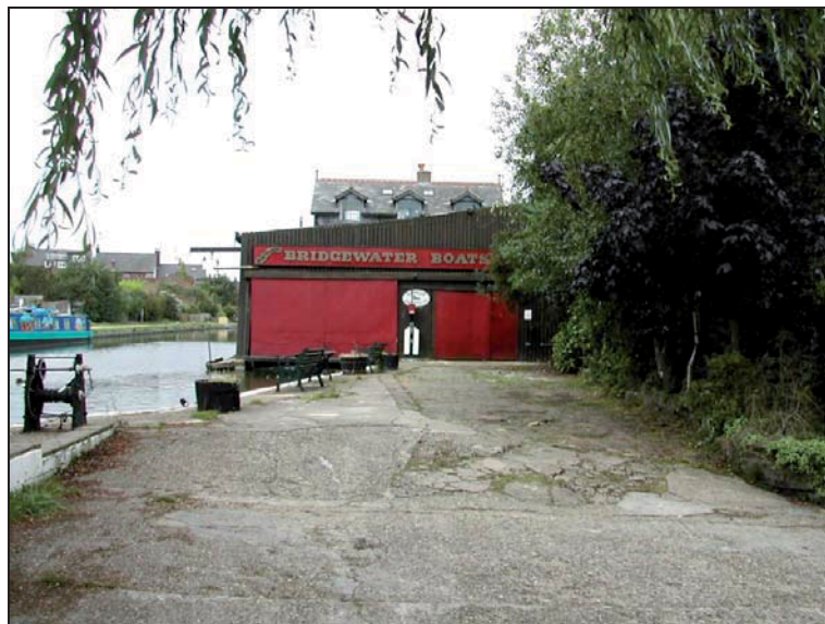
Plate 4: 'Bridgewater Boats' boat shed & concrete wharf looking SE
