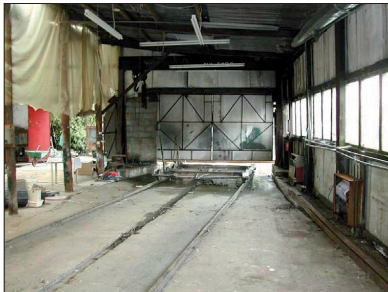
Plate 5: Interior of boat shed
