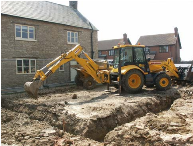
Plate 1: General view looking south
