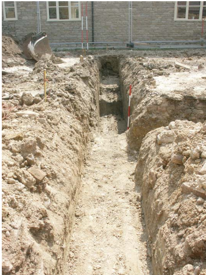
Plate 3: View south-westwards along the easternmost trench
