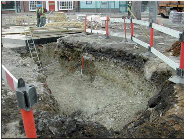
Plate 1: View north into foundation of water channel
