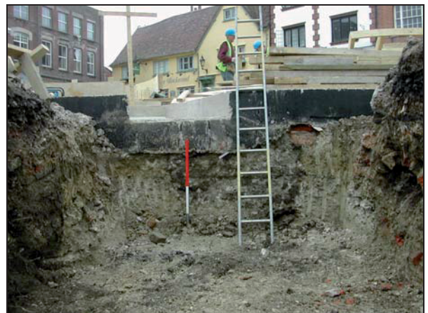
Plate 4: View north showing foundation of main water tank
