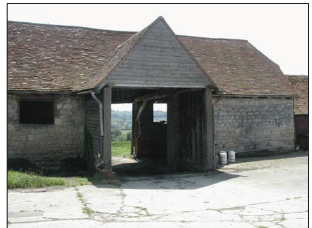
Plate 6: North facing elevation
