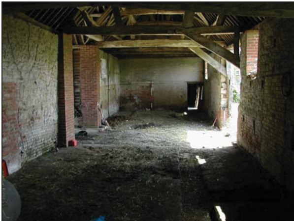
Plate 3: Interior of barn before work commenced
