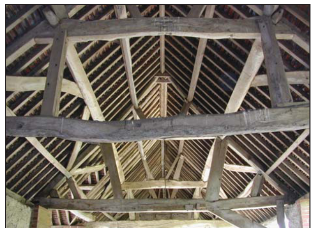
Plate 12: Detail of roof
