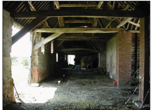
Plate 4: Interior view west
