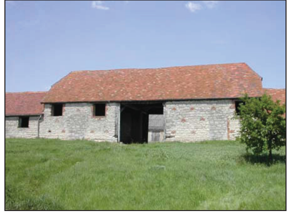
Plate 2: South facing external elevation
