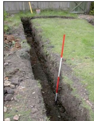
Plate 4: Southern E-W foundation
