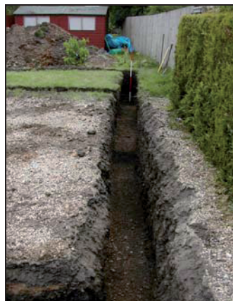
Plate 5: Western N-S foundation
