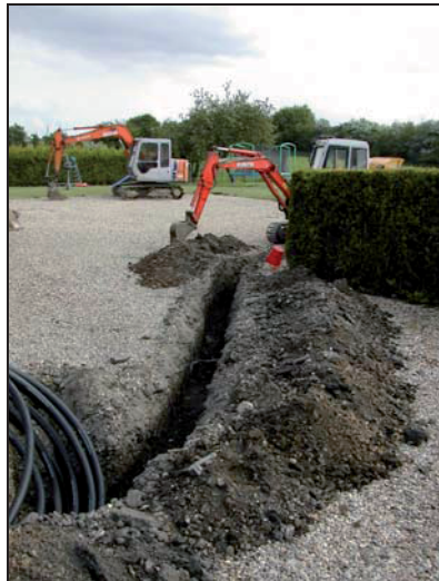
Plate 9: Service trench looking south
