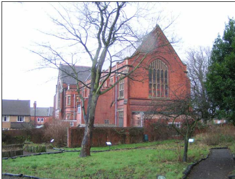
Plate 7: View of the north of the site with Fearon Hall in the background
