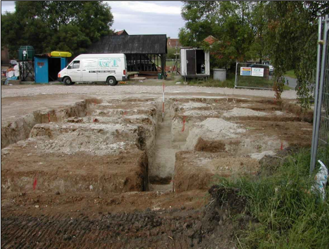
Plate 3: Foundation trenches of Plot 1 after excavation
