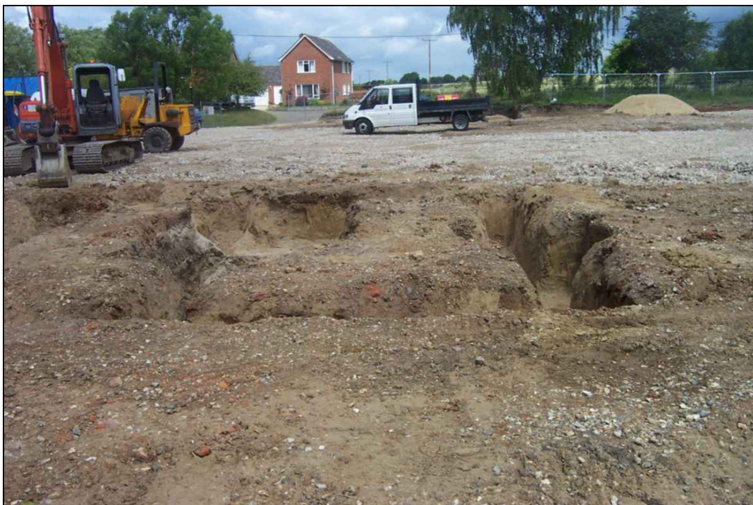
Plate 4: Foundation trenches of Plot 3 after excavation
