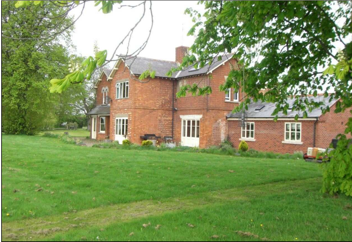
Plate 8: Caldecote Farmhouse, from south-east
