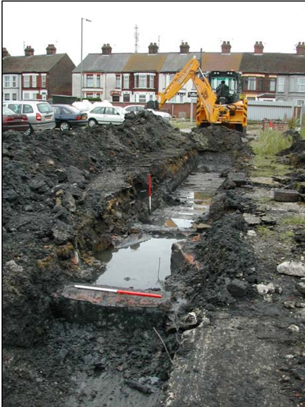
Plate 5: View SE showing foundations
