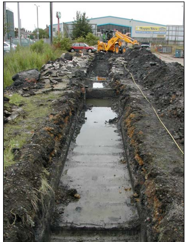
Plate 8: View NW showing trench extension
