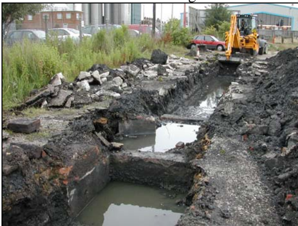
Plate 7: View NW showing character of foundations
