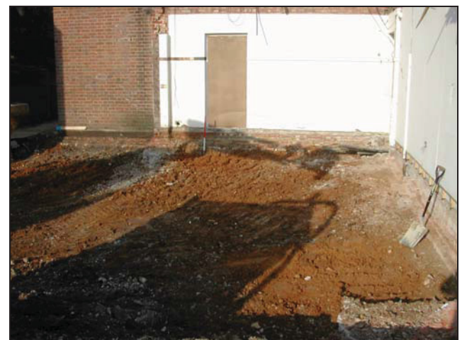
Plate 6: Detail of sub-soils beneath northern building extension
