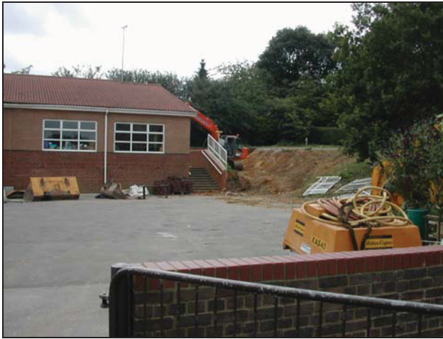
Plate 1: View south to the southern building extension
