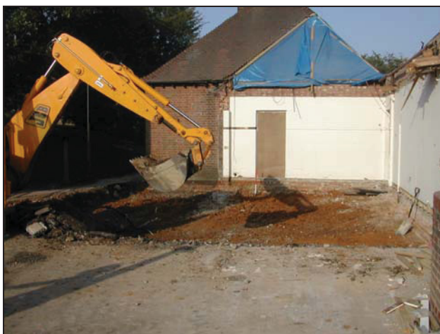
Plate 5: View west across area of northern building extension
