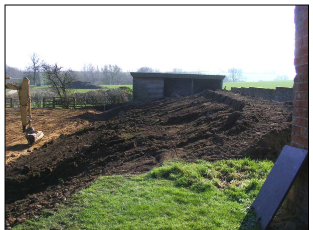
Plate 6: Bank fully excavated and sloped, looking south
