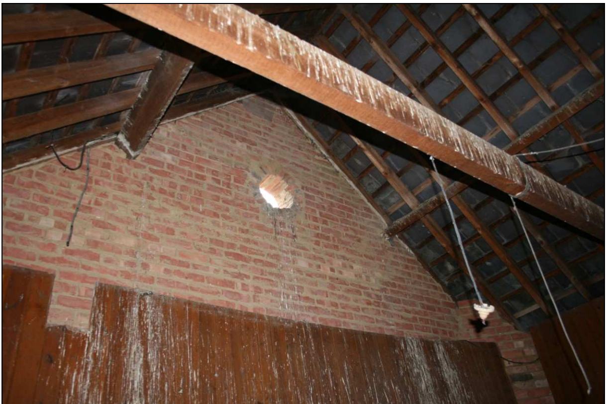
Plate 9: Building 2, Room 1, east gable looking south-east
