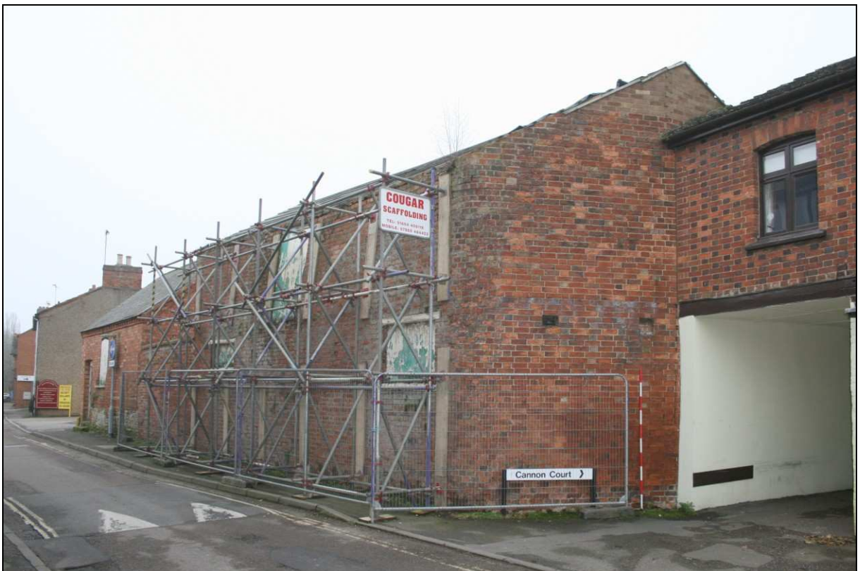
Plate 2: Building 1, Union Street frontage from north-west
