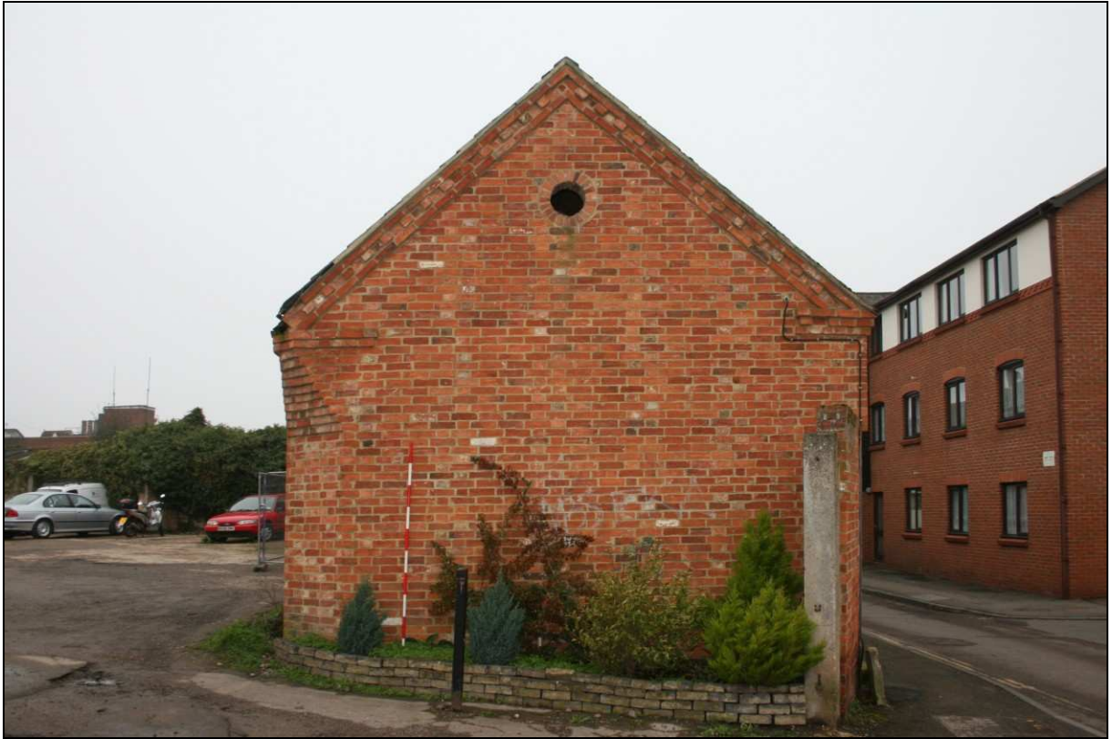
Plate 5: Building 2, east elevation from east
