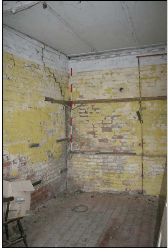
Plate 11: Building 2, Room 2, looking north
