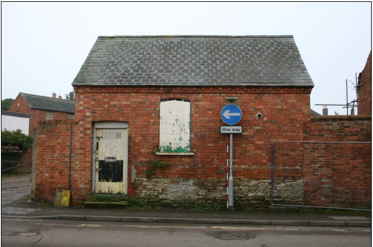
Plate 6: Building 2, north elevation from north
