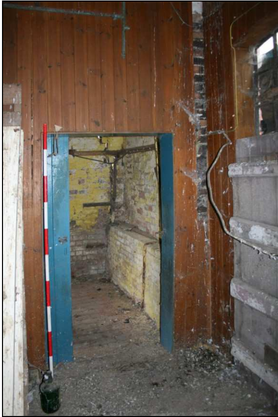
Plate 10: Building 2, Room 1, doorway to Room 2
