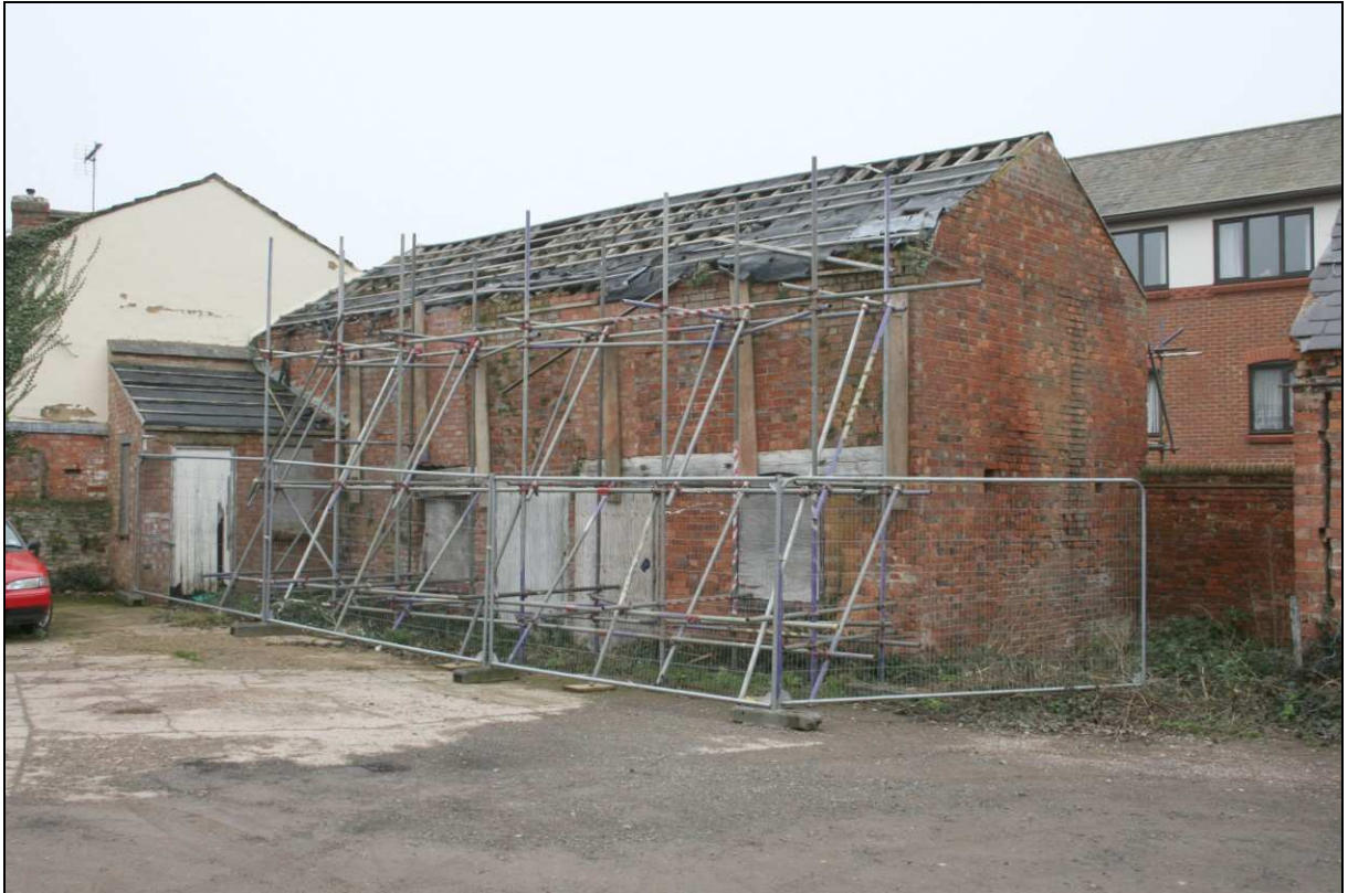
Plate 1: Building 1, south elevation from south-east
