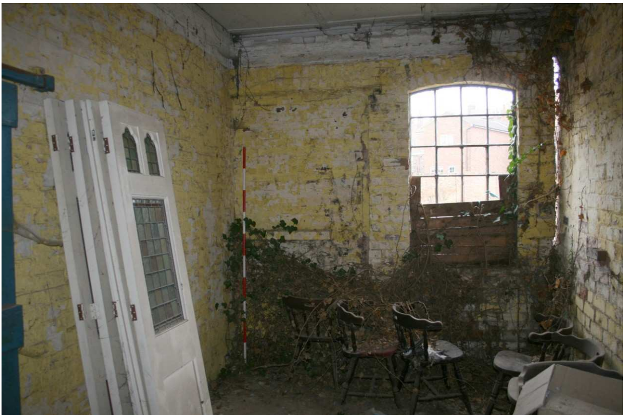
Plate 12: Building 2, Room 2, looking south
