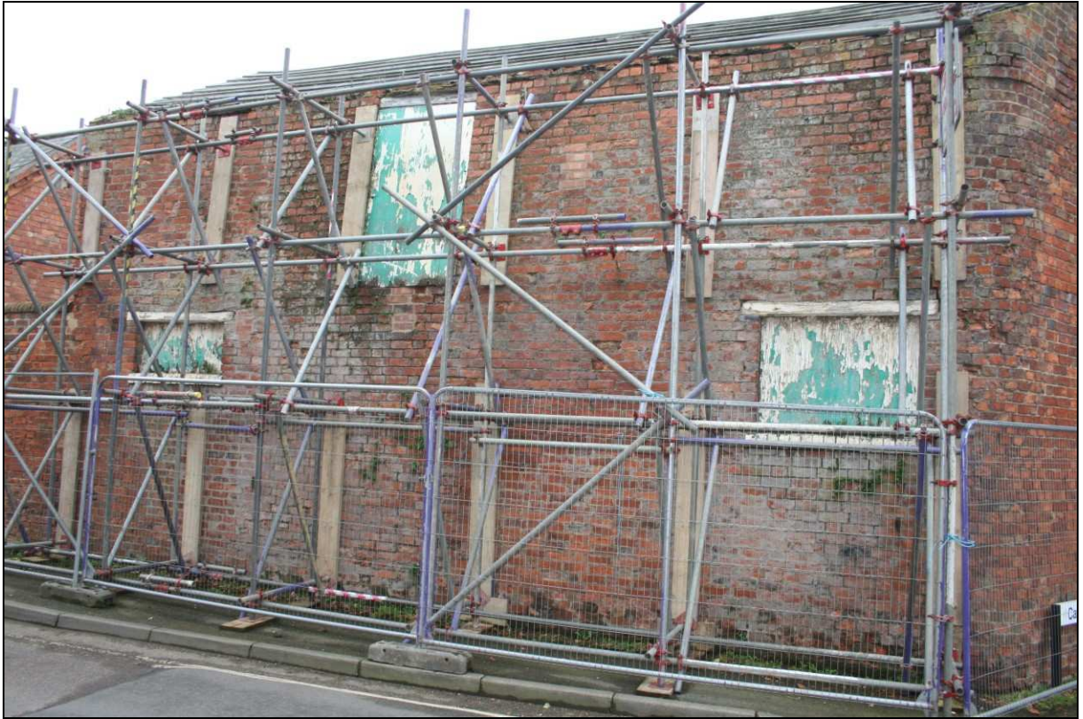
Plate 3: Building 1, north elevation from north
