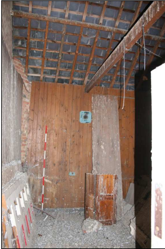
Plate 7: Building 2, Room 1, looking south
