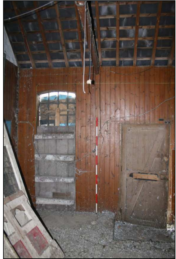
Plate 8: Building 2, Room 1, looking north
