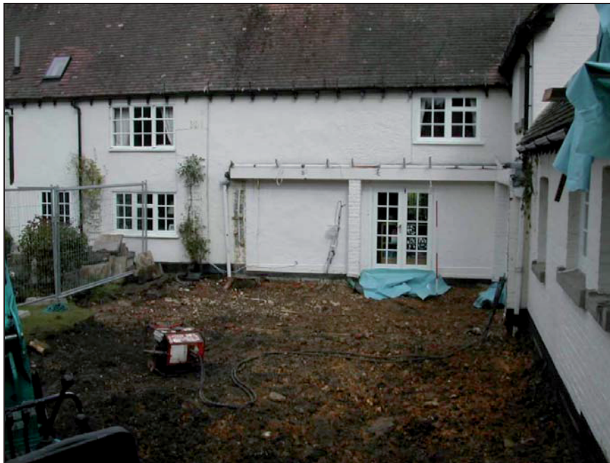
Plate 1: The footprint of the new extension
