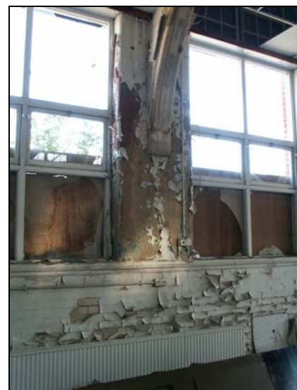
Plate 54: [12], north wall, structural detail
