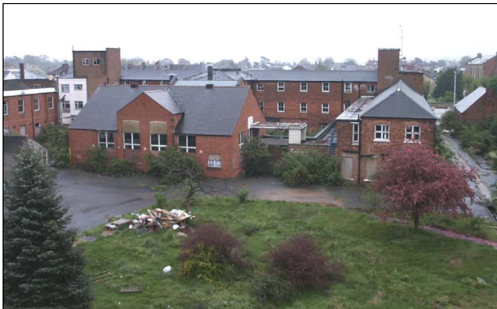
General view of main workhouse complex, from infirmary Buildings, left to right: [15], [12] ([01f] and Hub to rear), [01e], [13], [02]
