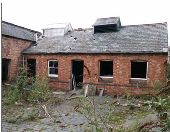
Plate 23: [04], south elevation, central wing
