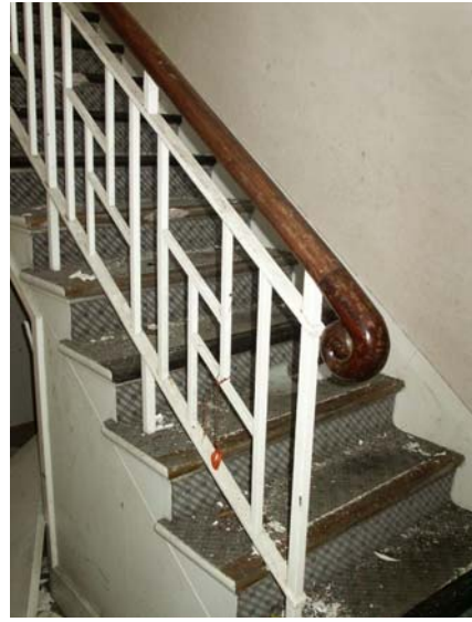
Plate 32: [06], detail of stairs
