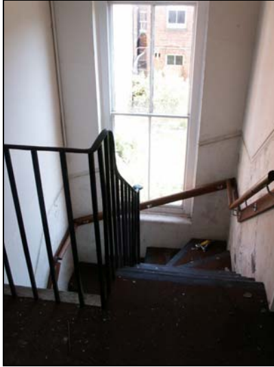
Plate 7: [01d], second floor, stairwell
