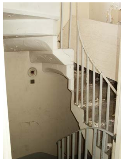
Plate 12: [01f], first floor, stairwell
