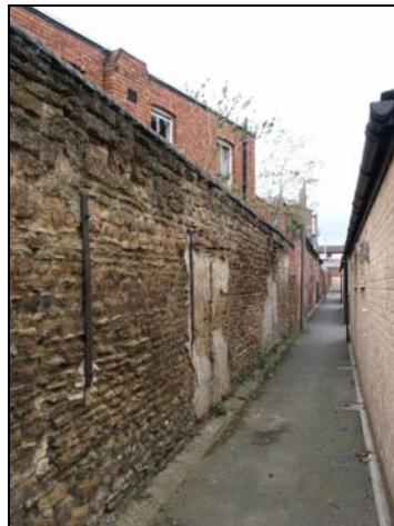
Plate 63: Stone boundary wall, east side of site
