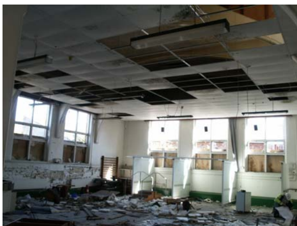
Plate 53: [12], interior looking NE
