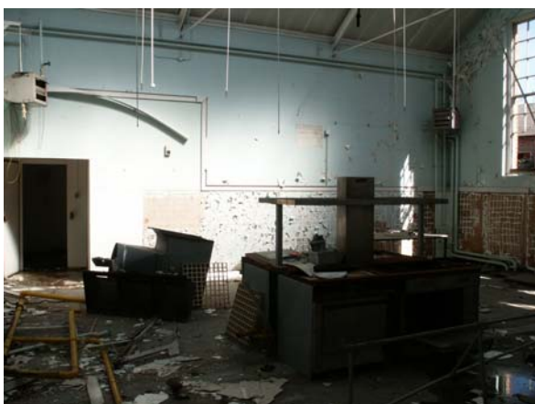
Plate 59: [14], interior, looking NE
