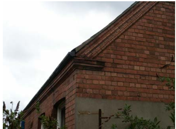
Plate 20: [02], detail of north gable end
