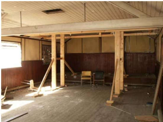
Plate 45: [10], first floor looking north
