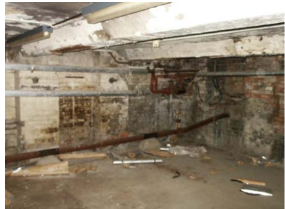
Plate 40: [08], cellar, SE corner
